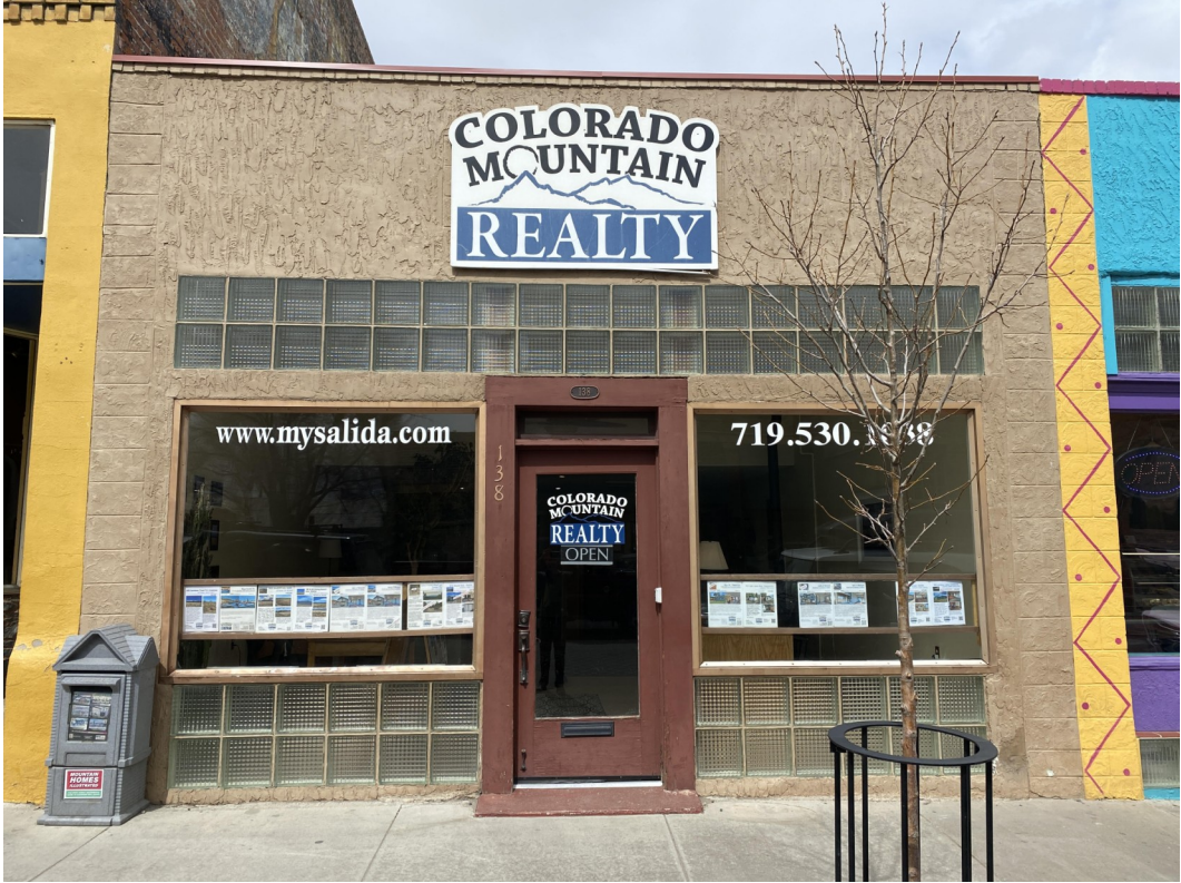
Existing Storefront / 138 North F Street
