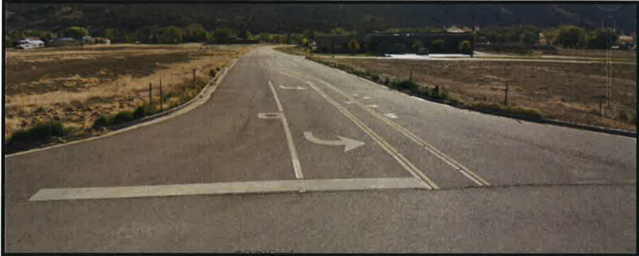
Figure 9-Vandaveer Ranch Road looking East from Highway 50
