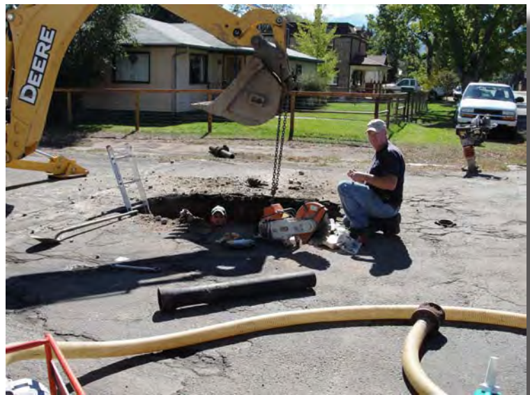
Public Works Repairing Water Lines
