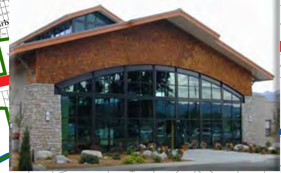
Salida Hot Springs Aquatic Center
