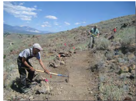
Salida Mountain Trails- Frontside Trail being built by local volunteers
