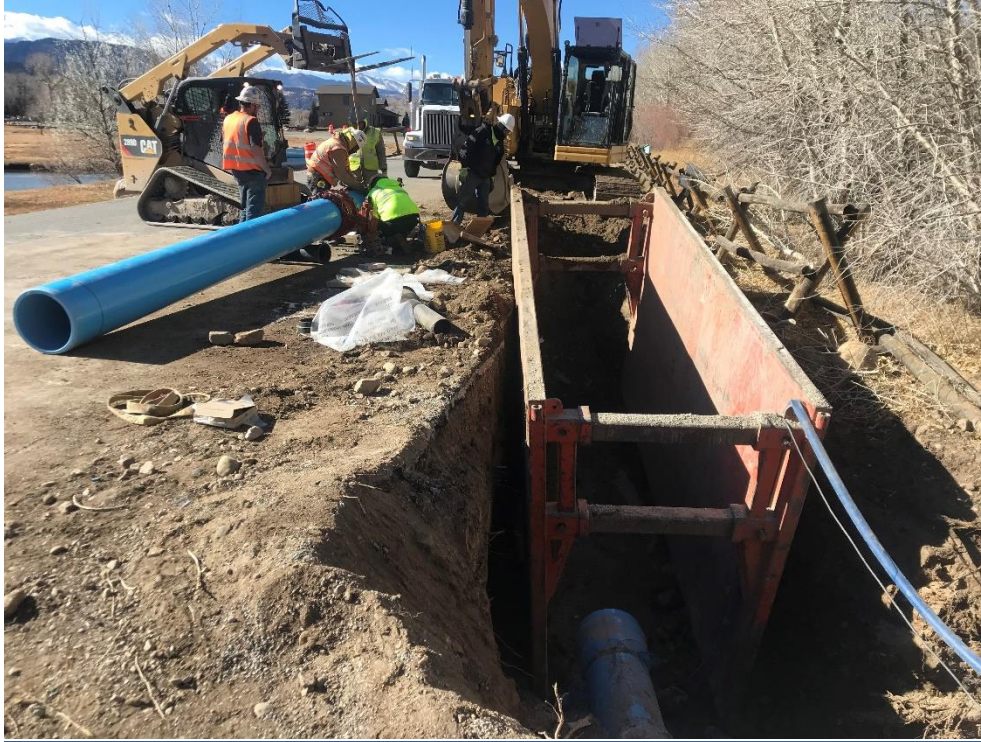
Figure 1- Low Zone Waterline Replacement Project
