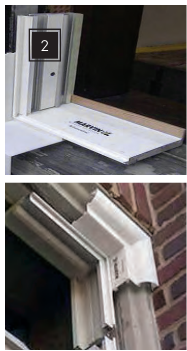
SIDE JAMB VERTICAL MULL Note: Detail shows the relationship of the daylight opening to the brick. Special sized stile and rail components might be required to match both the glass DLO and the brick to DLO dimensions.
