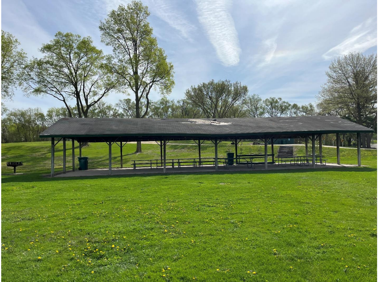
Riverside Park Pavilion
