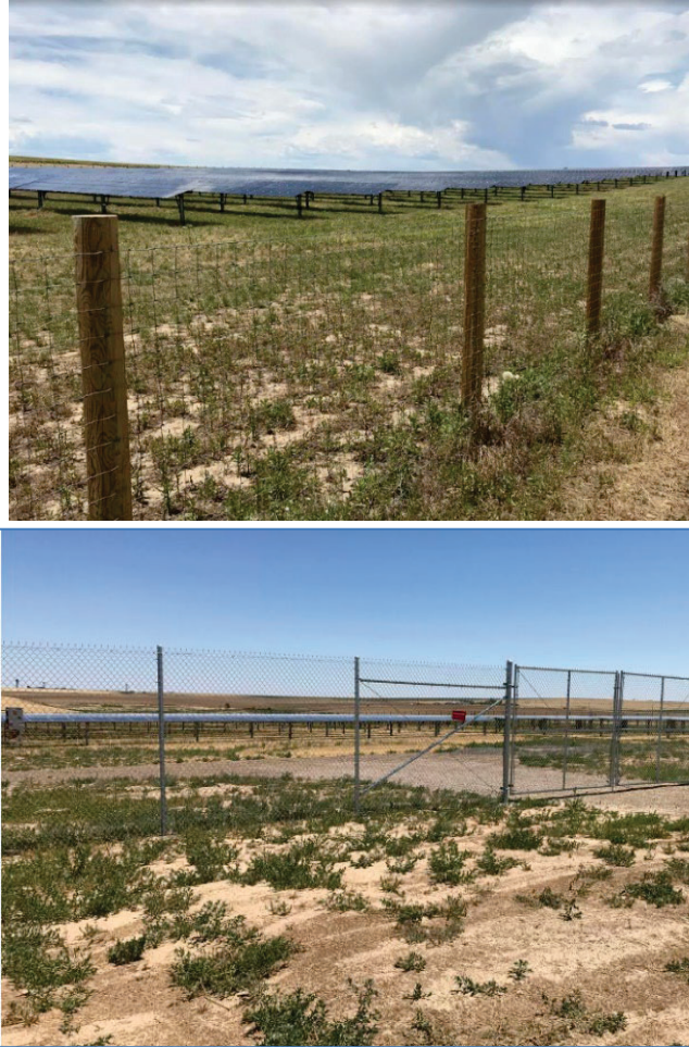
Photo 3. Depiction of the difference between agricultural style fencing (left) and chain link (right).
