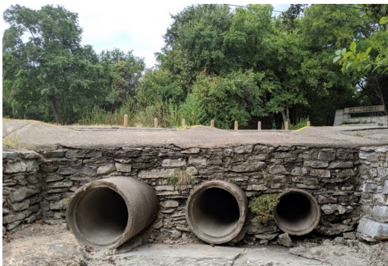
Figure 1: Edgegrove Drive Low Water Crossing (September 11, 2019)
