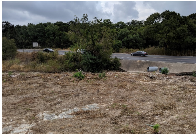
Figure 5: Bee Caves Road Culvert, Downstream (September 11, 2019)
