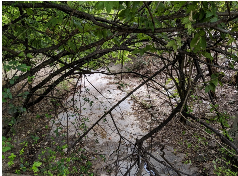
Figure 6: Rockway Cove Culvert, Looking Southwest/Upstream (September 11, 2019)
