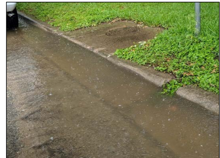
Pond inlet during rain event. 06/06/2019
