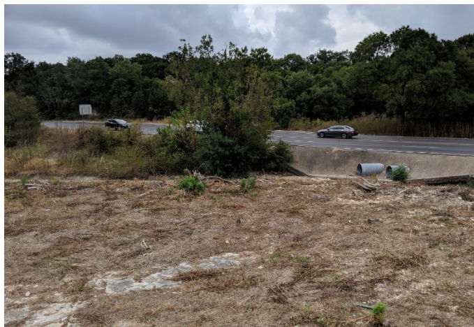
Figure 5: Bee Caves Road Culvert, Downstream (September 11, 2019)
