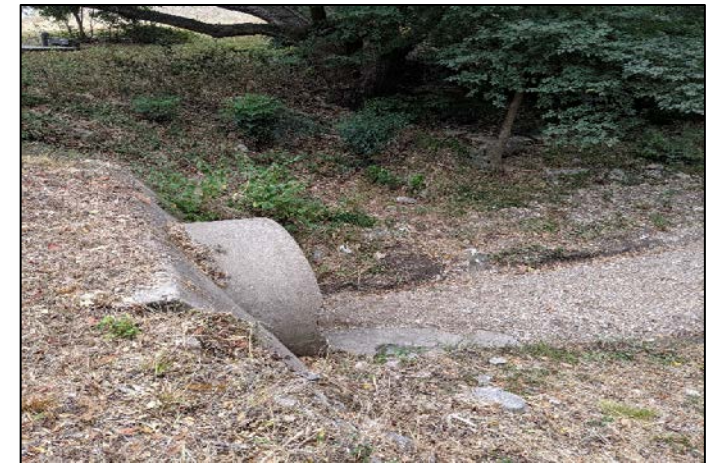
Pleasant Cove culvert crossing, upstream. 09/11/2019
