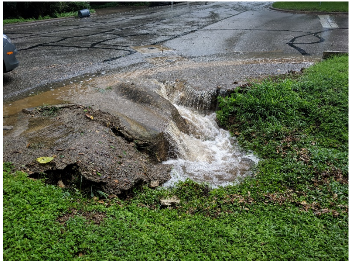
Figure 4: Nixon Drive Culvert, Looking Southeast/Downstream (June 6, 2019)
