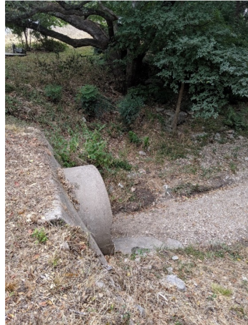
Figure 7: Pleasant Cove Culvert, Looking Northeast/Downstream (September 11, 2019)
