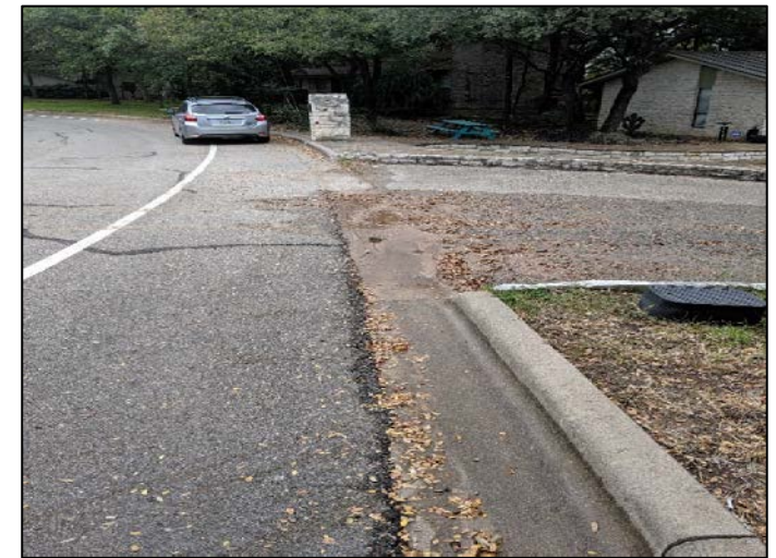
Timberline Drive looking northeast. 09/11/2019
