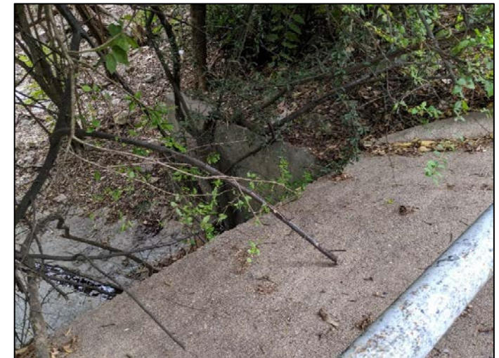
Outfall at Town Lake tributary. 09/11/2019
