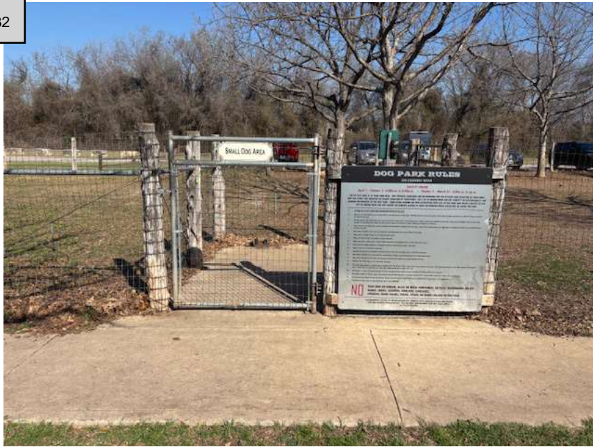
Double gated entrance with concrete paving
