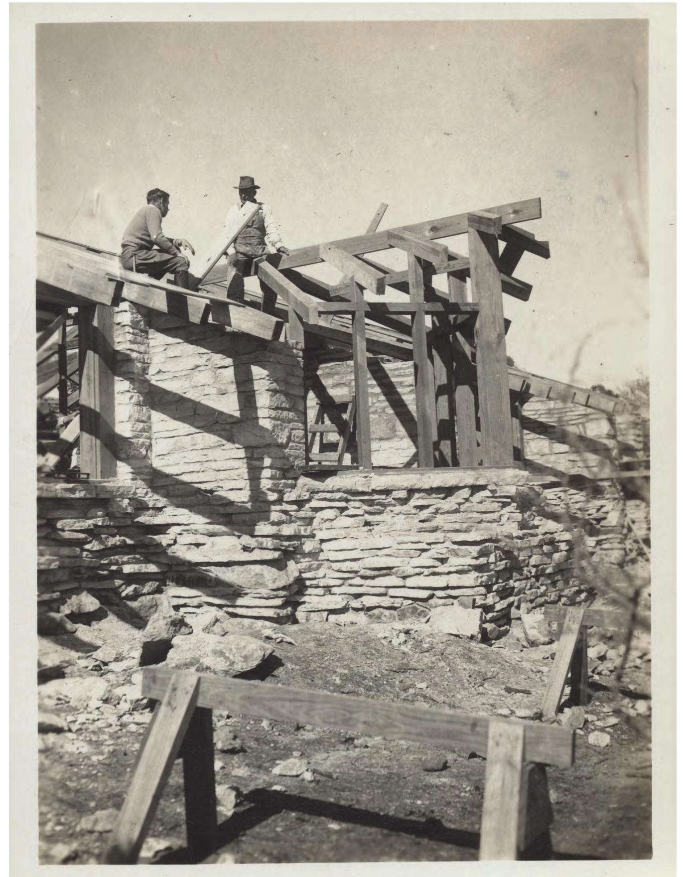
Boy Scout Clubhouse construction, ca. 1934, Austin History Center
