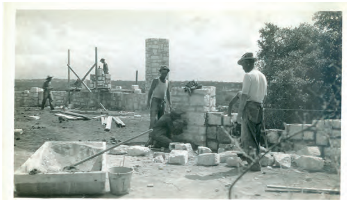
Lookout Point construction, 1934, Austin History Center
