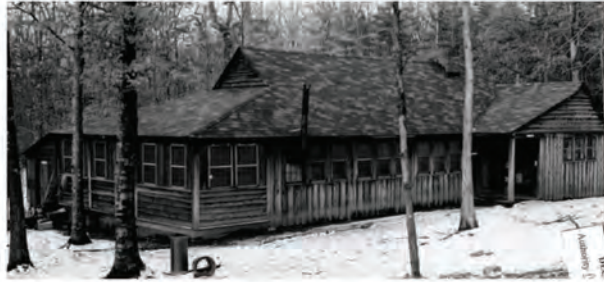
This 1945 image of the Camp 4 Craft Lodge shows the OSS added asphalt shingles. National Archives and Records Administration
