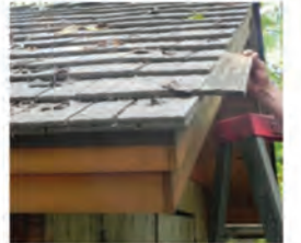
A worker holds up a original cedar shake to the roof of a cabin covered in the chosen composite material
