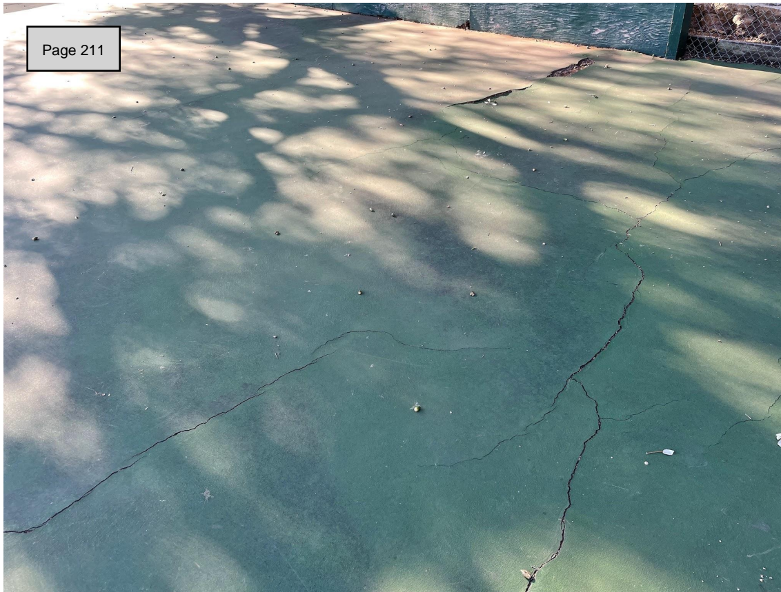
Lower court damage : multiple cracks (some dangerous), worn surface
