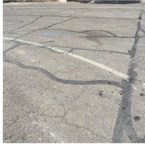
Timberline Dr PCI Rating = 66 Fair Strategy: Mill and Overlay
