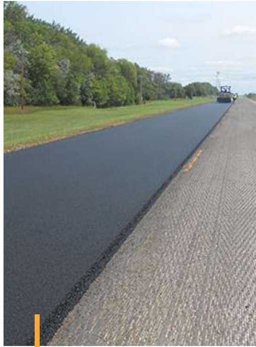
Mill and Overlay Typical for Fair Rated Roadways
