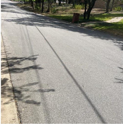
Almarion Way PCI Rating = 92 Excellent Strategy: Creak sealing
