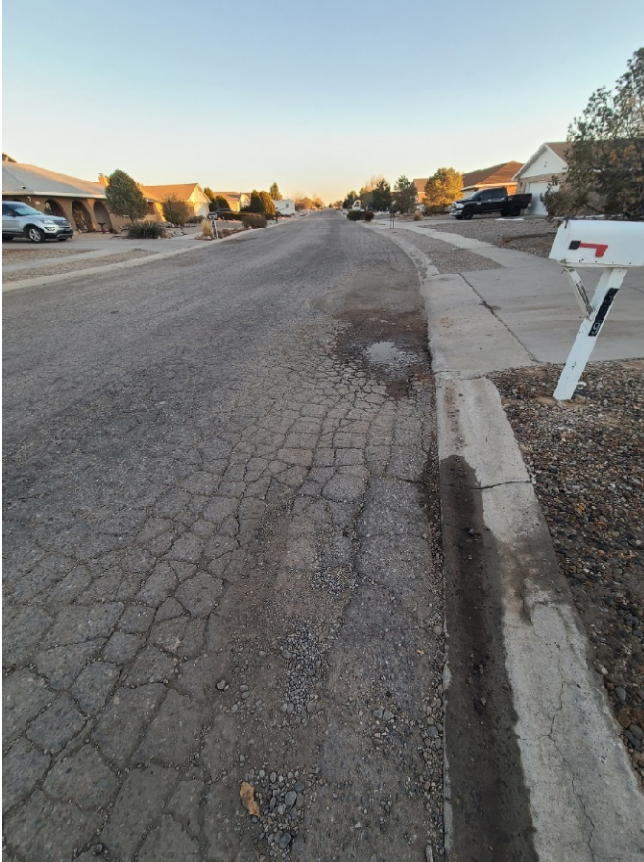
Figure 3: Alligator cracking
