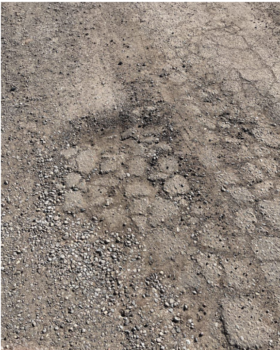
Figure 4: Alligator cracking and subgrade failure
