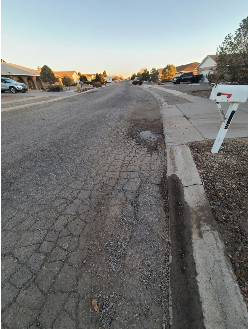
Figure 3: Alligator cracking
