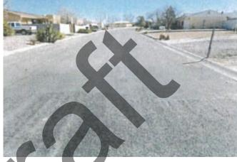
**Repair:** Chip-seal **Area:** 60,000 SF (W30' X L2,000')
