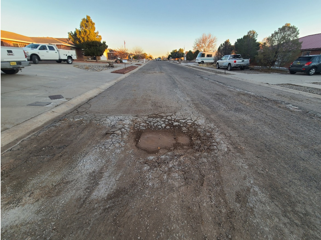
Figure 1: Subgrade exposure
