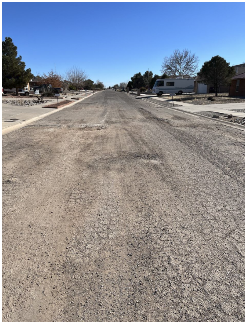
Figure 2: Excessive cracking and subgrade exposure
