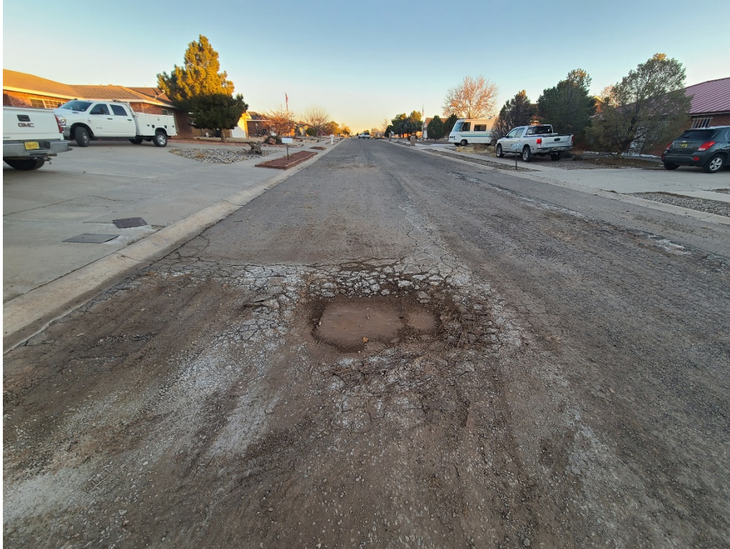
Figure 1: Subgrade exposure
