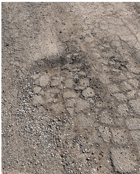
Figure 4: Alligator cracking and subgrade failure
