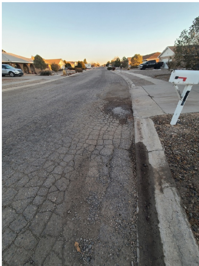
Figure 3: Alligator cracking
