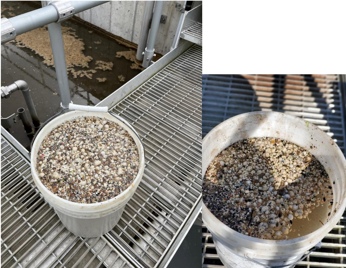
Grease balls floating at the top of the WWTP and collected 04/26/2023
