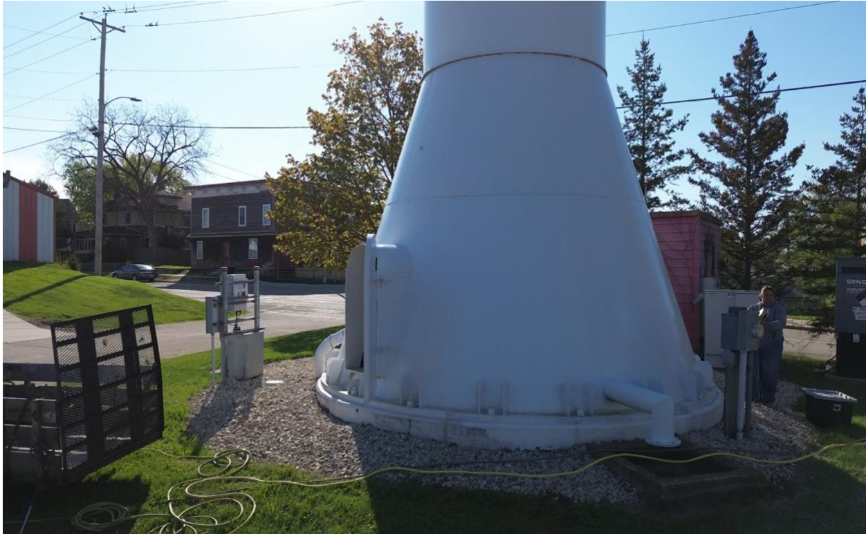
Base Cone Before Power Washing
