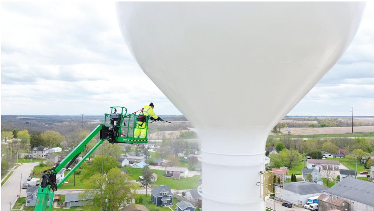
Worker Power Washing to Remove Dirt and Mildew
