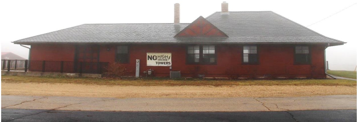
AHI No. 64662, Chicago and Northwestern Depot, rear (south) elevation, facing north. The existing parking lot adjacent to the depot, in the foreground, will be repaved as a result of the project.
