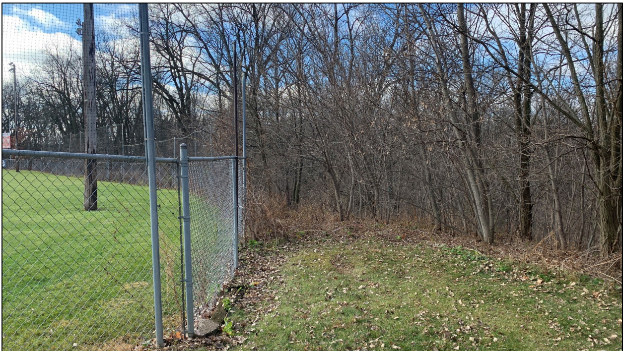
Figure 6. Northern corner of the baseball field, near the foul ball pole along the first baseline, view west. Note the drop off almost immediately adjacent to the fence in the background. Photo taken 11/11/22.
