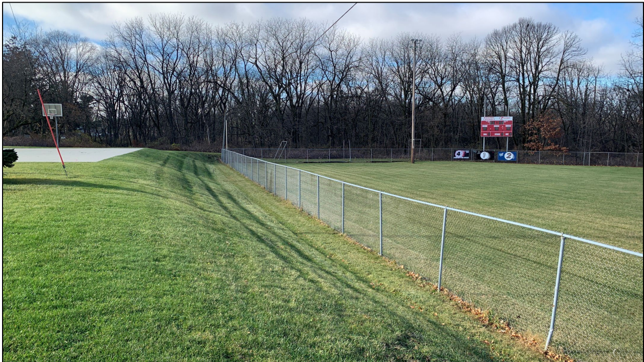
Figure 4. Southern side of the baseball field showing shaped area, view southwest. Photo taken 11/11/22.
