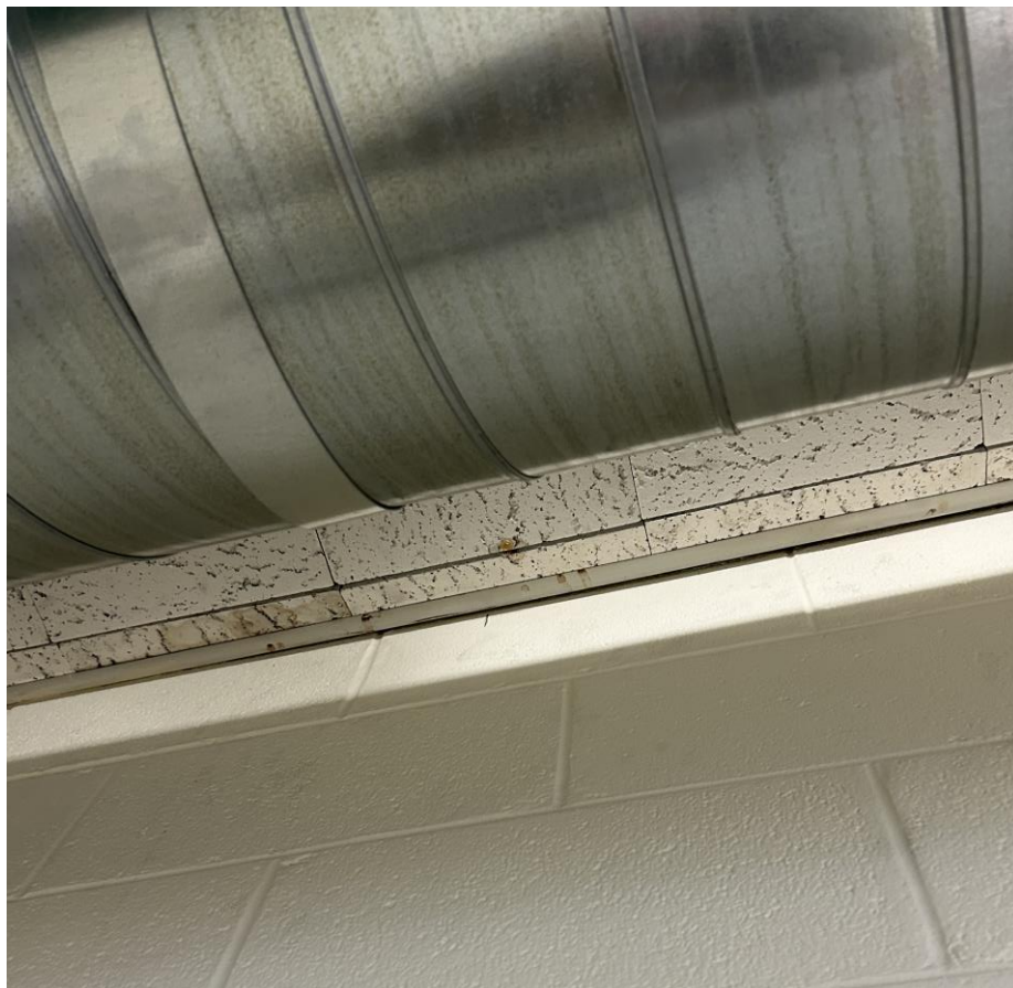
CEILING AND HALLWAY ACROSS FROM LIBRARY
