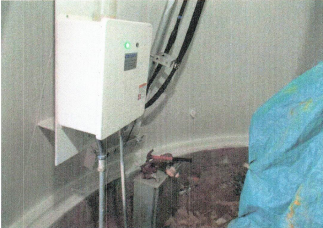
Interior Dry Base Bell - Good Condition
