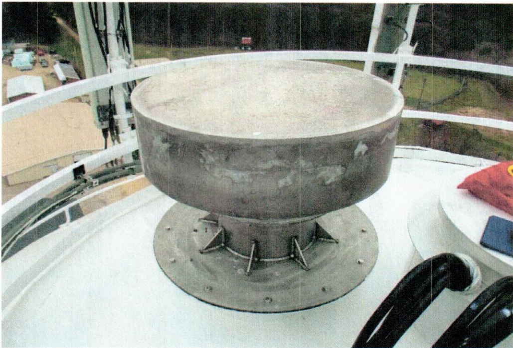
Exterior Roof Vent - Good Condition
