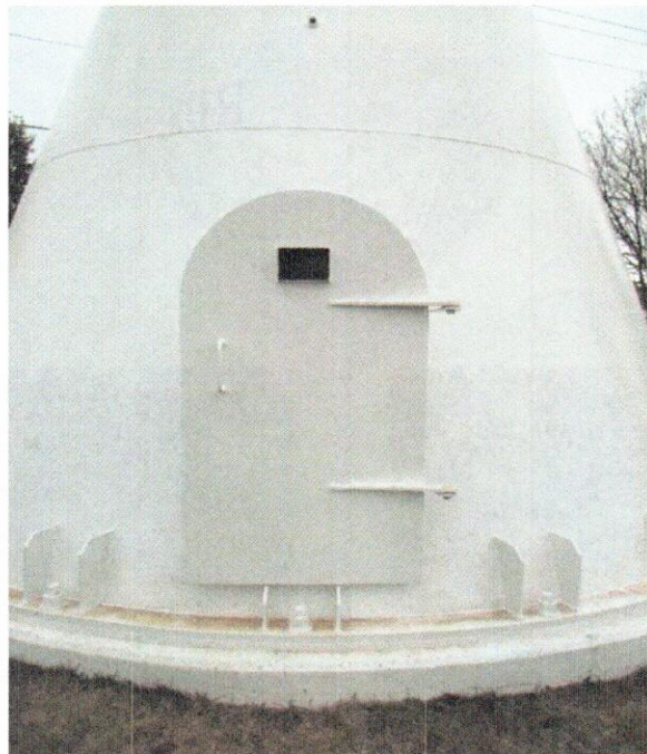
Exterior Door – Good Condition
