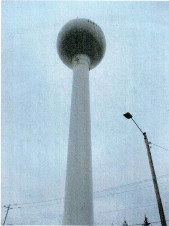
Exterior Riser - Good Condition
