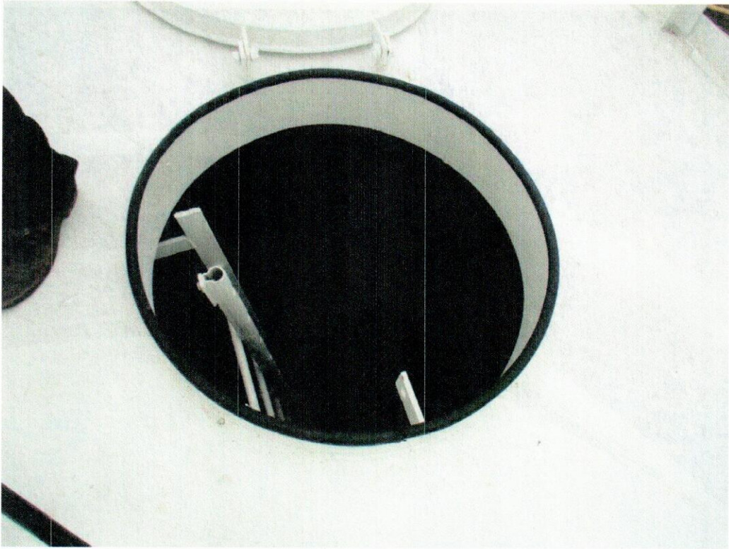
Exterior Wet Hatch - Good Condition
