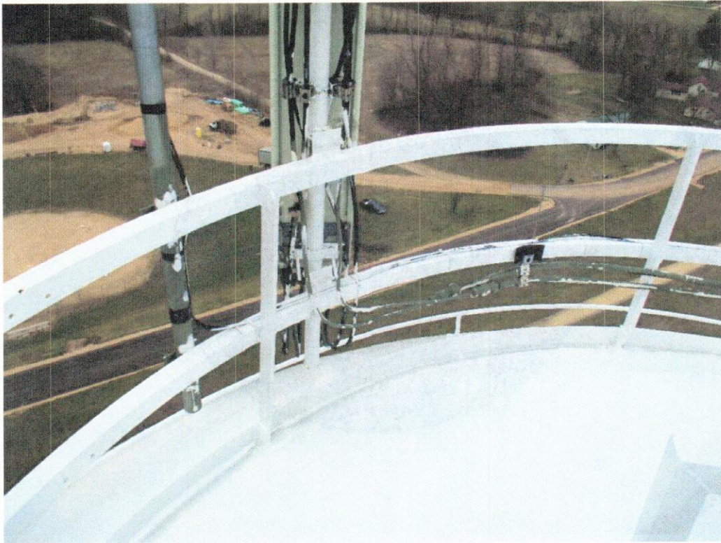
Exterior Roof and Handrail – Good Condition
