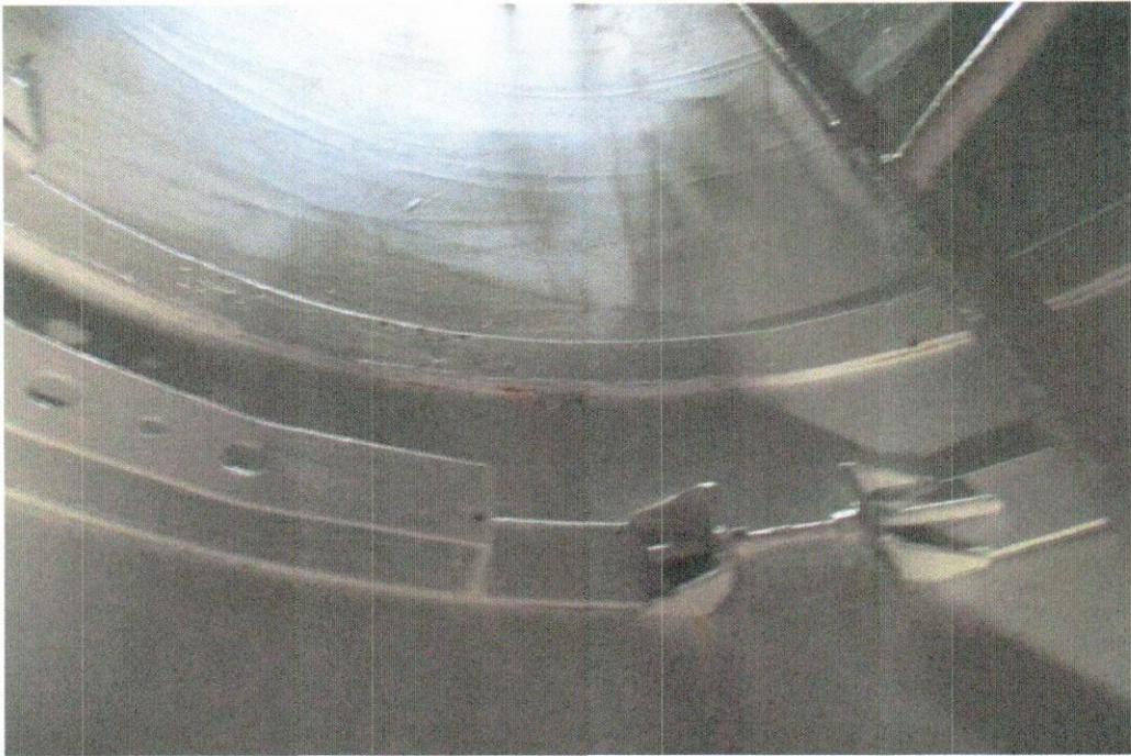
Access Tube – Good Condition
