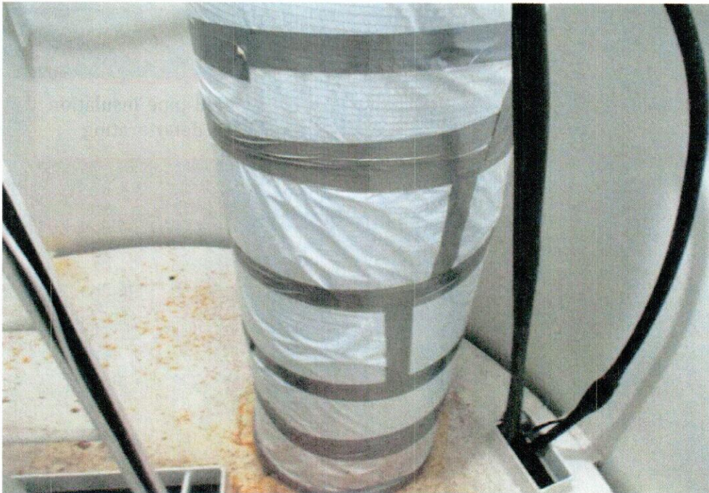
Top Platform - Good Condition - Minor Staining
