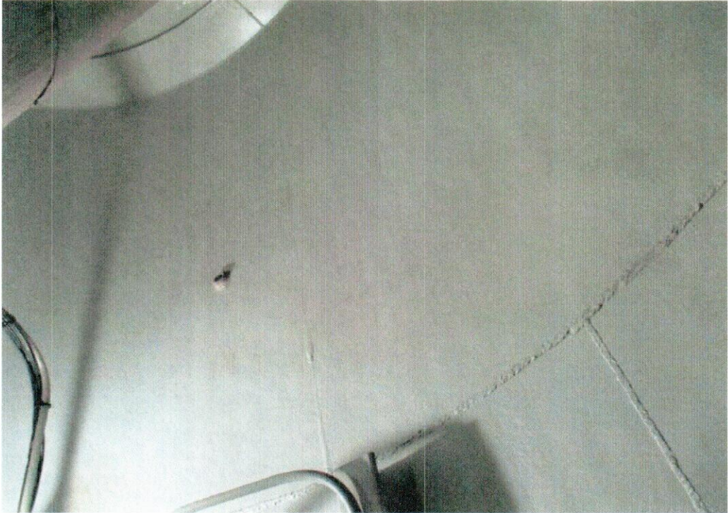
Interior Dry Base Bell - Good Condition
