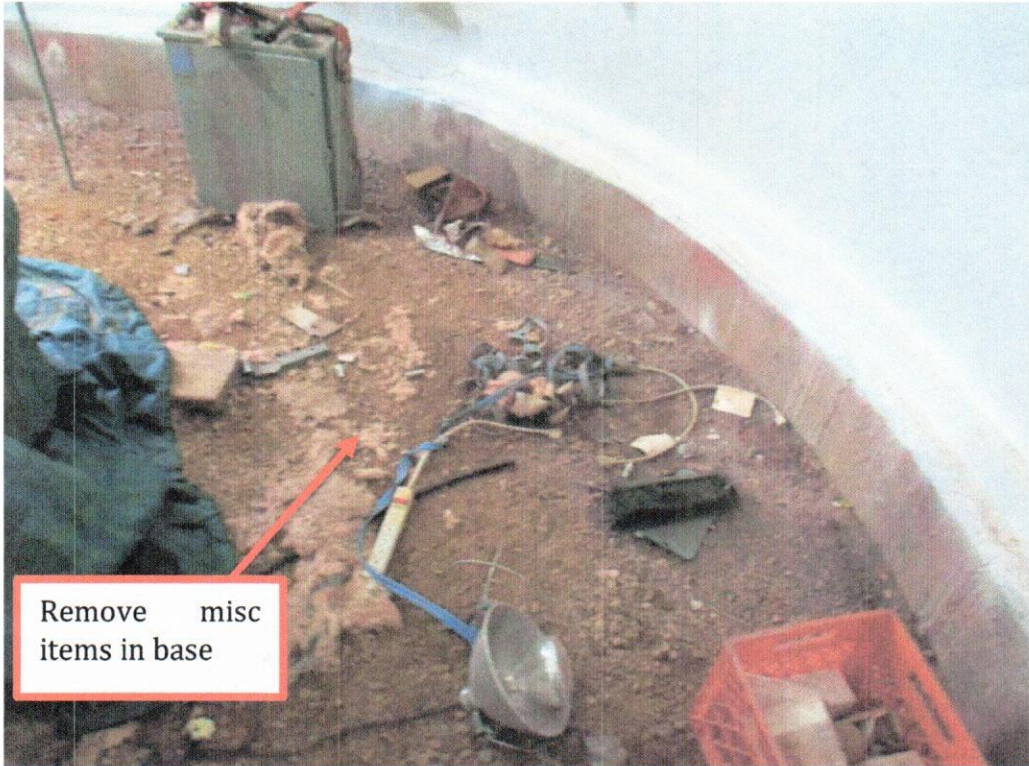
Interior Dry Base Bell - Miscellaneous Cables and Debris Left in Tank
