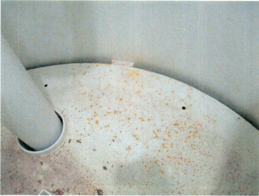
Top Platform - Good Condition - Minor Debris and Staining
