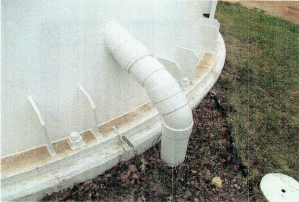
Exterior Foundation - Good Condition
