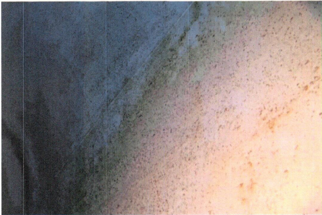
Interior Wet Sidewalls – Good Condition – Minor Staining
