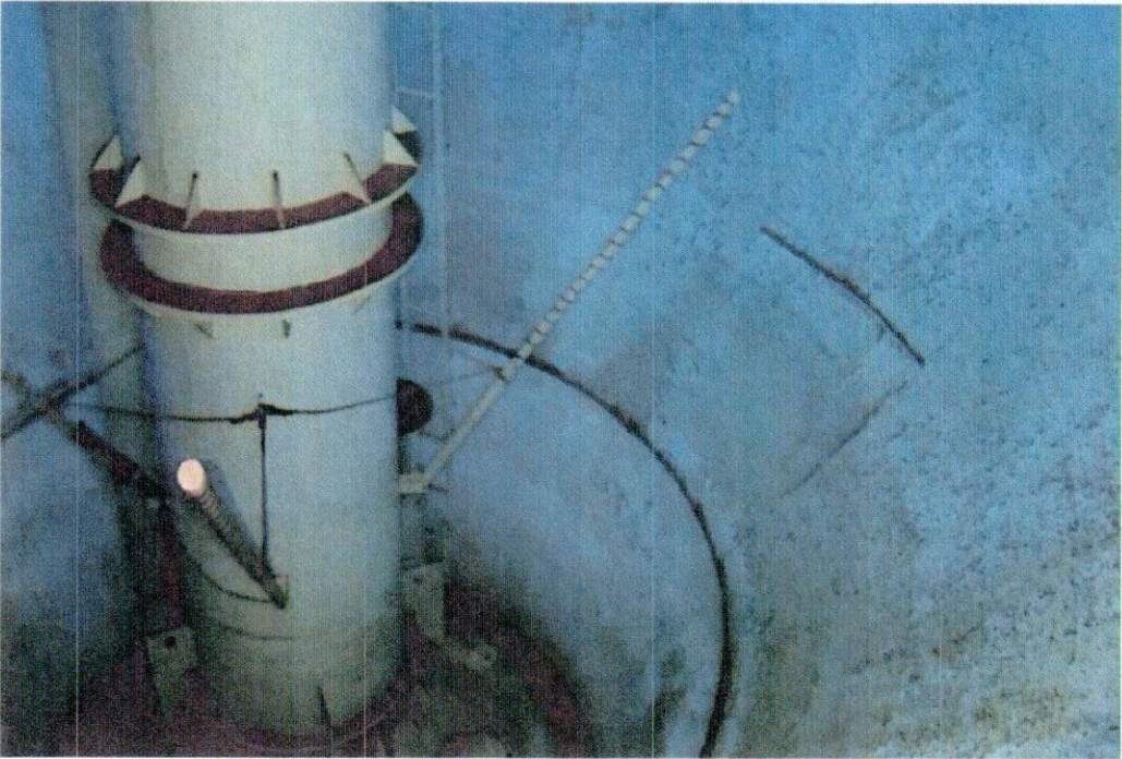
Interior Wet - Good Condition - Minor Sediment
