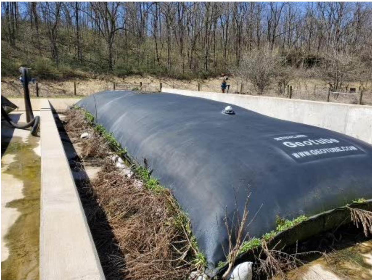
Picture #5 - Geotube Ready for Removal
