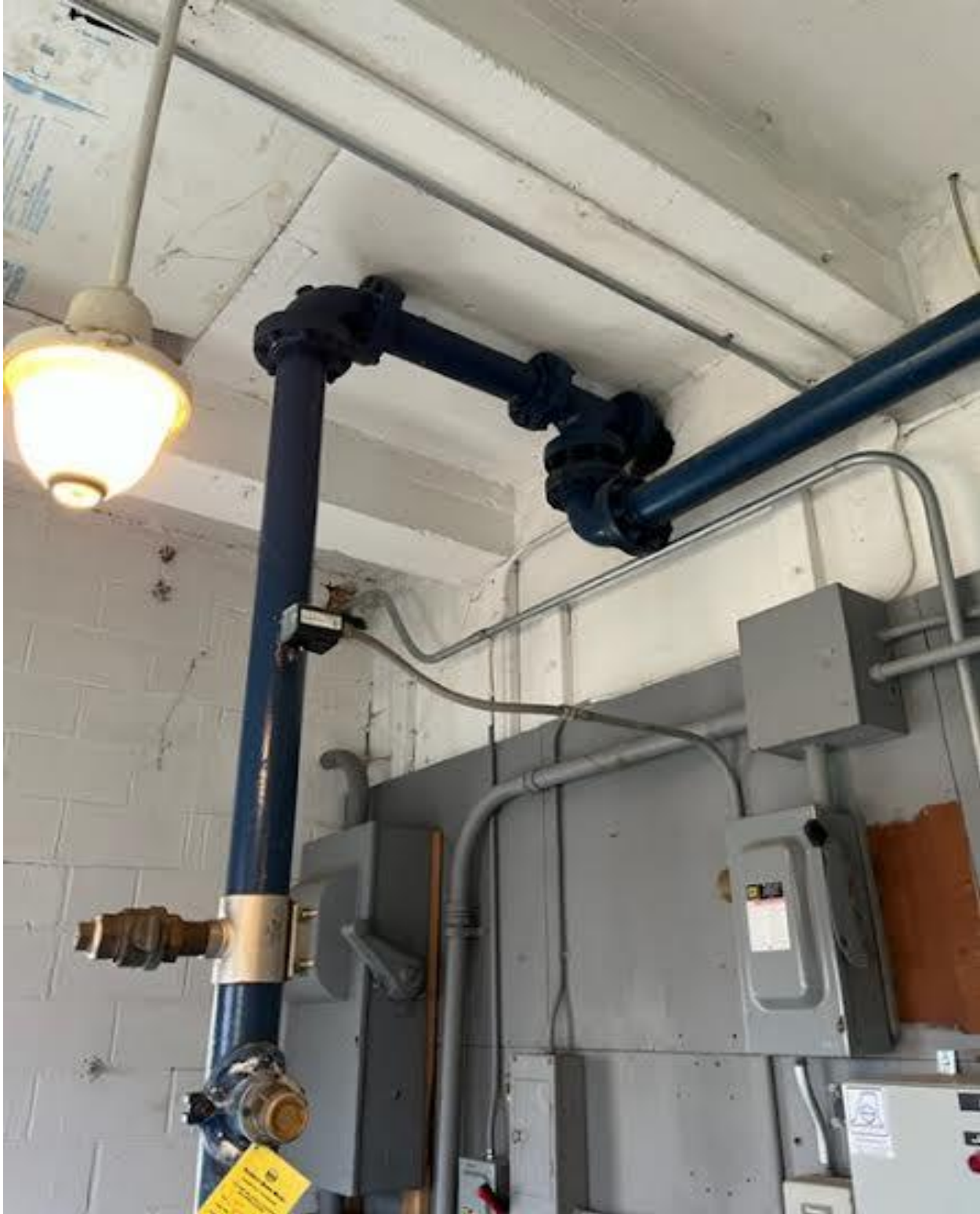
The Fill Pipe is in Good Condition
