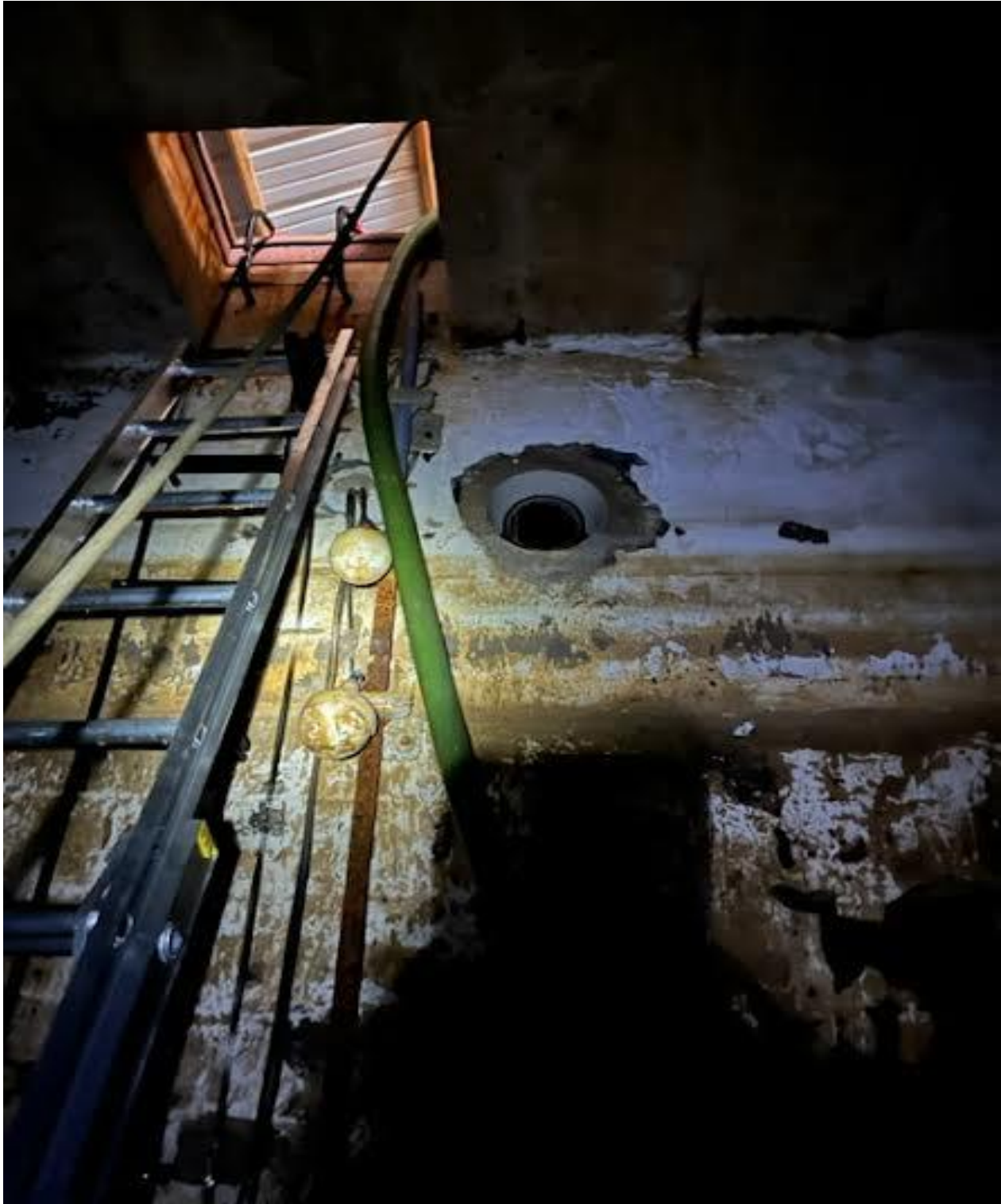
The Overflow Opening and Floats are in Good Condition
