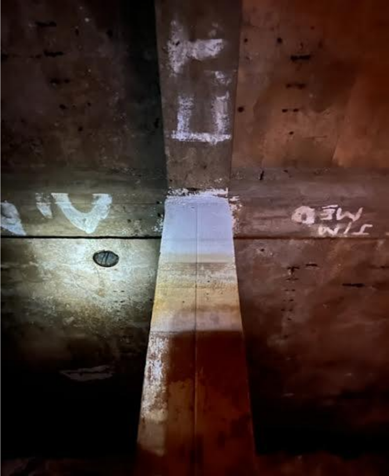
The Concrete Beams are in Good Condition
