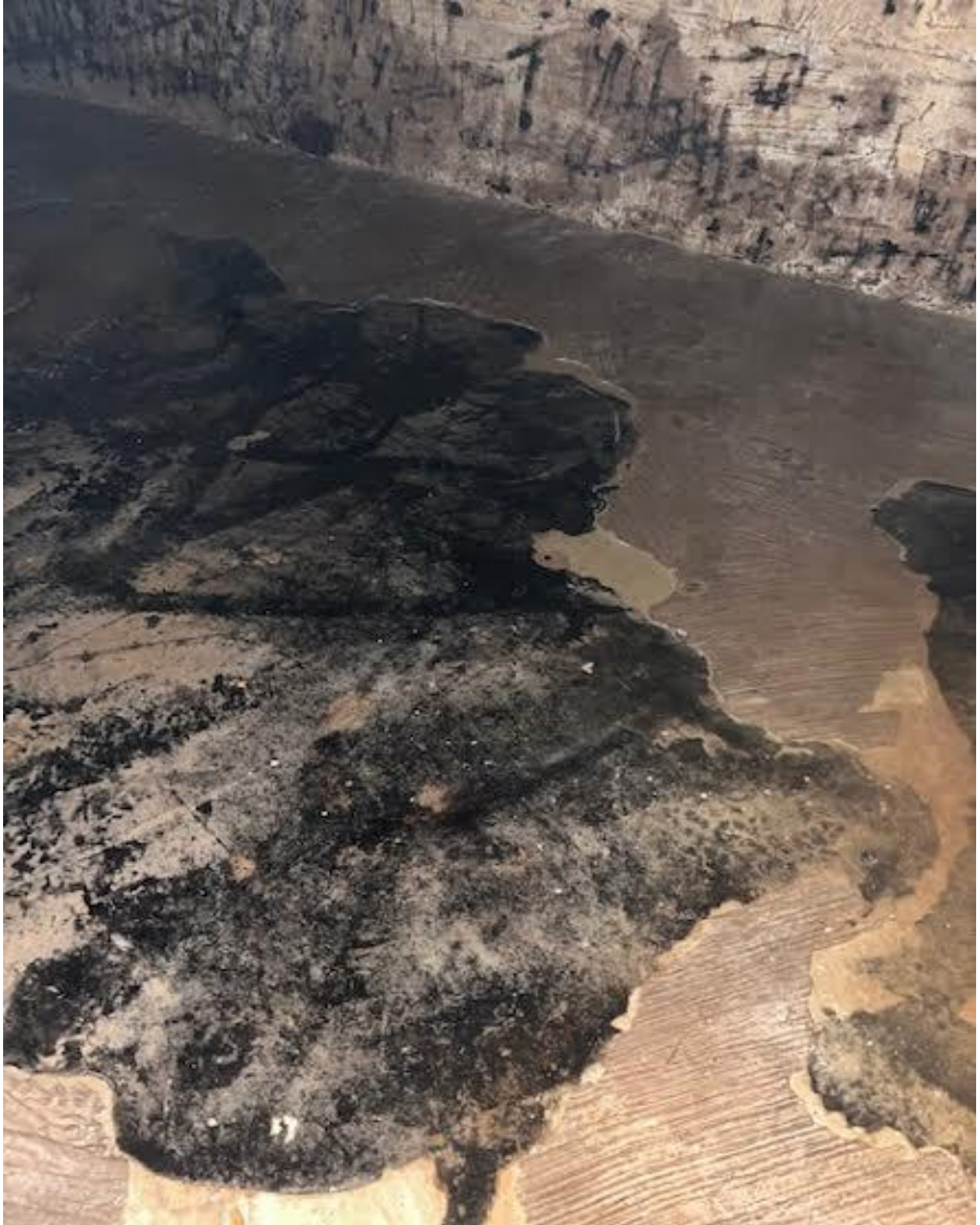
The Concrete Floor is in Good Condition
