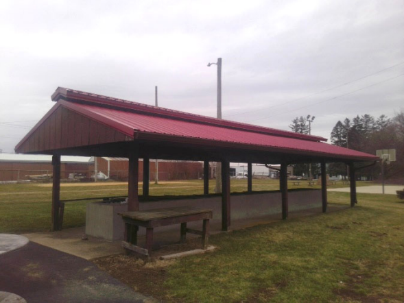
006003 - Picnic Shelter #1 (Exterior View)
