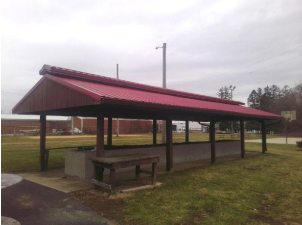
006003 - Picnic Shelter #1 (Exterior View)
