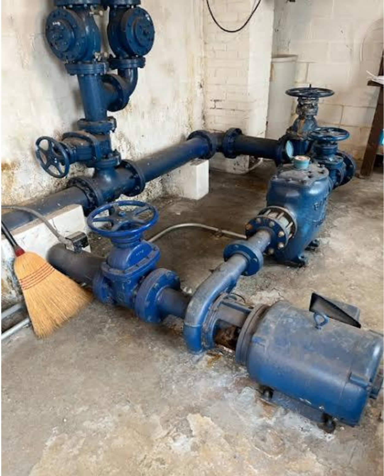
The Outlet Pipe is in Good Condition
