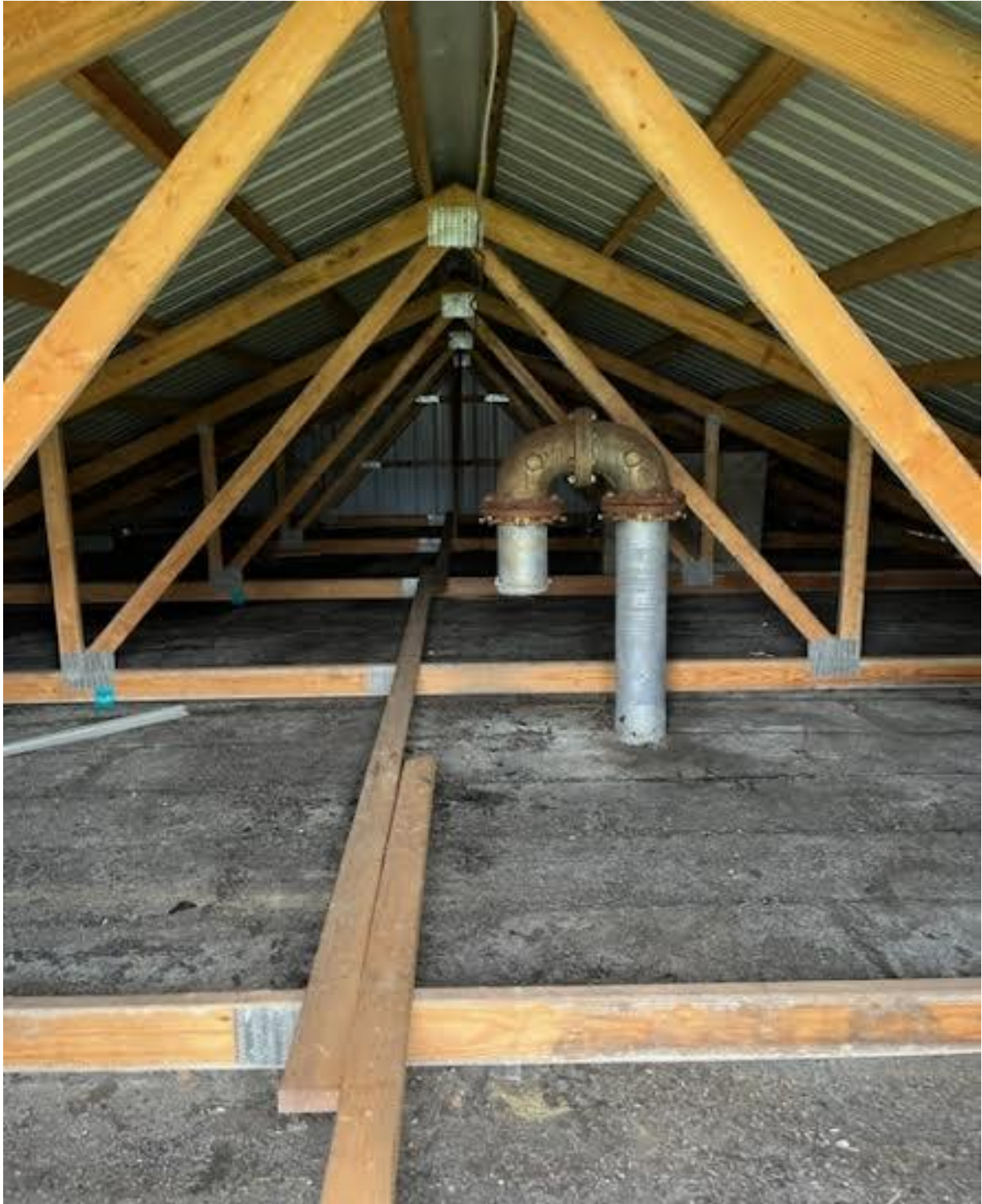
Metal Air Vent is in Good Condition
