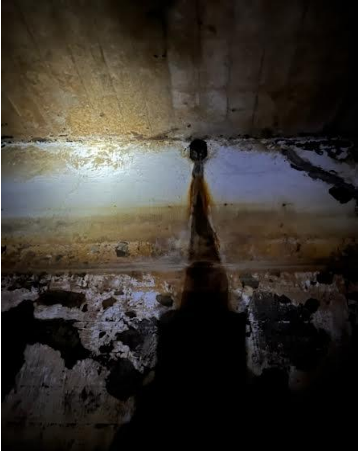
The Fill Pipe is in Good Condition
