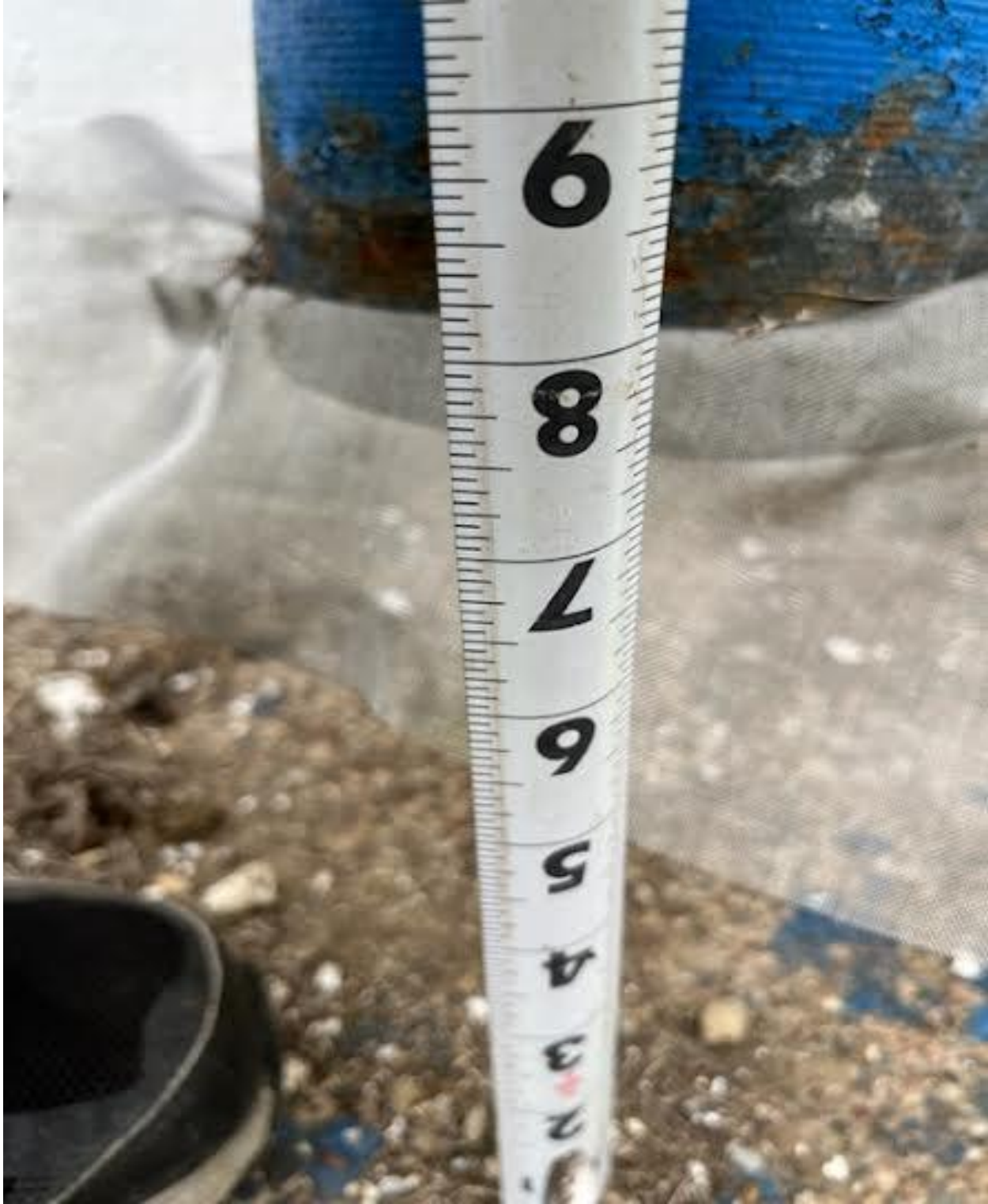
The Overflow Air Gap is at 8"
