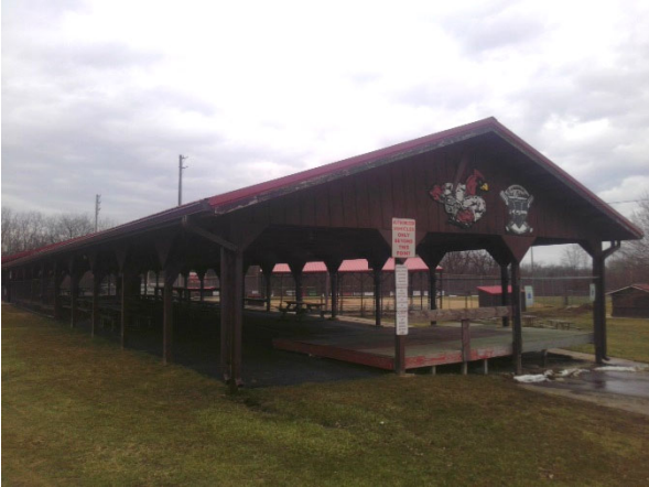
006004 - Picnic Shelter #2 (Exterior View)
