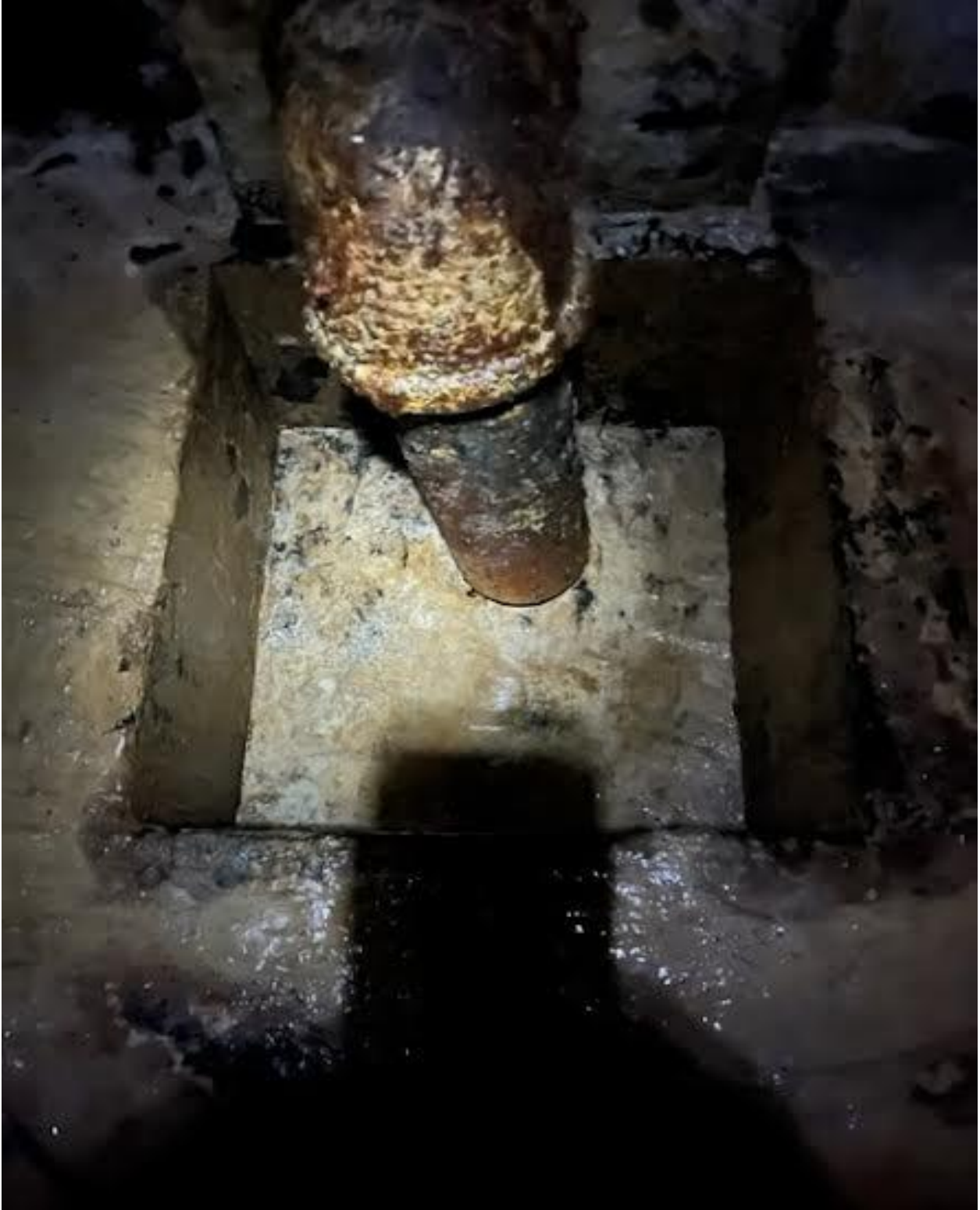
The Sump Area was Cleaned Out
