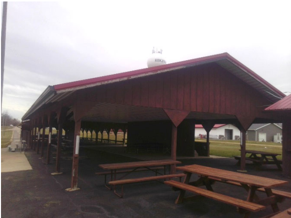
006005 - Picnic Shelter #3 (Exterior View)
