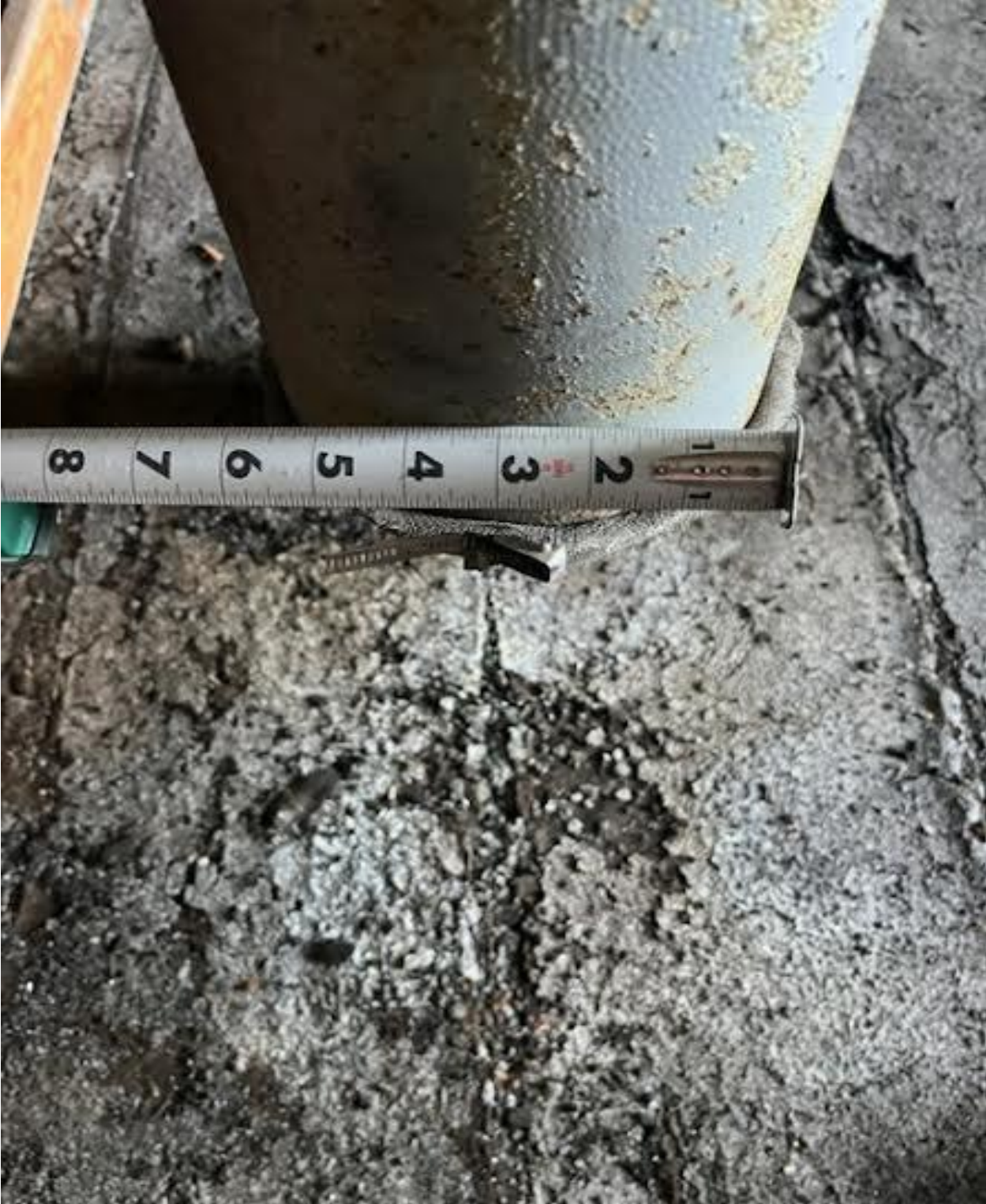
6" Diameter Air Vent
