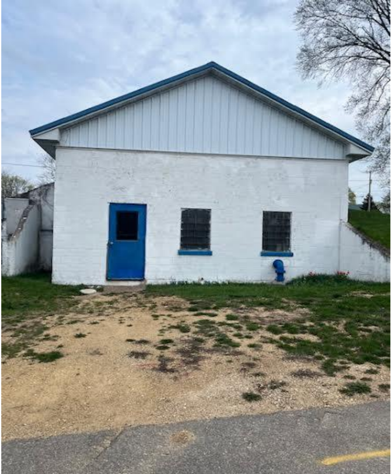
Well No #1 - 40,000 Gallon Concrete Reservoir
