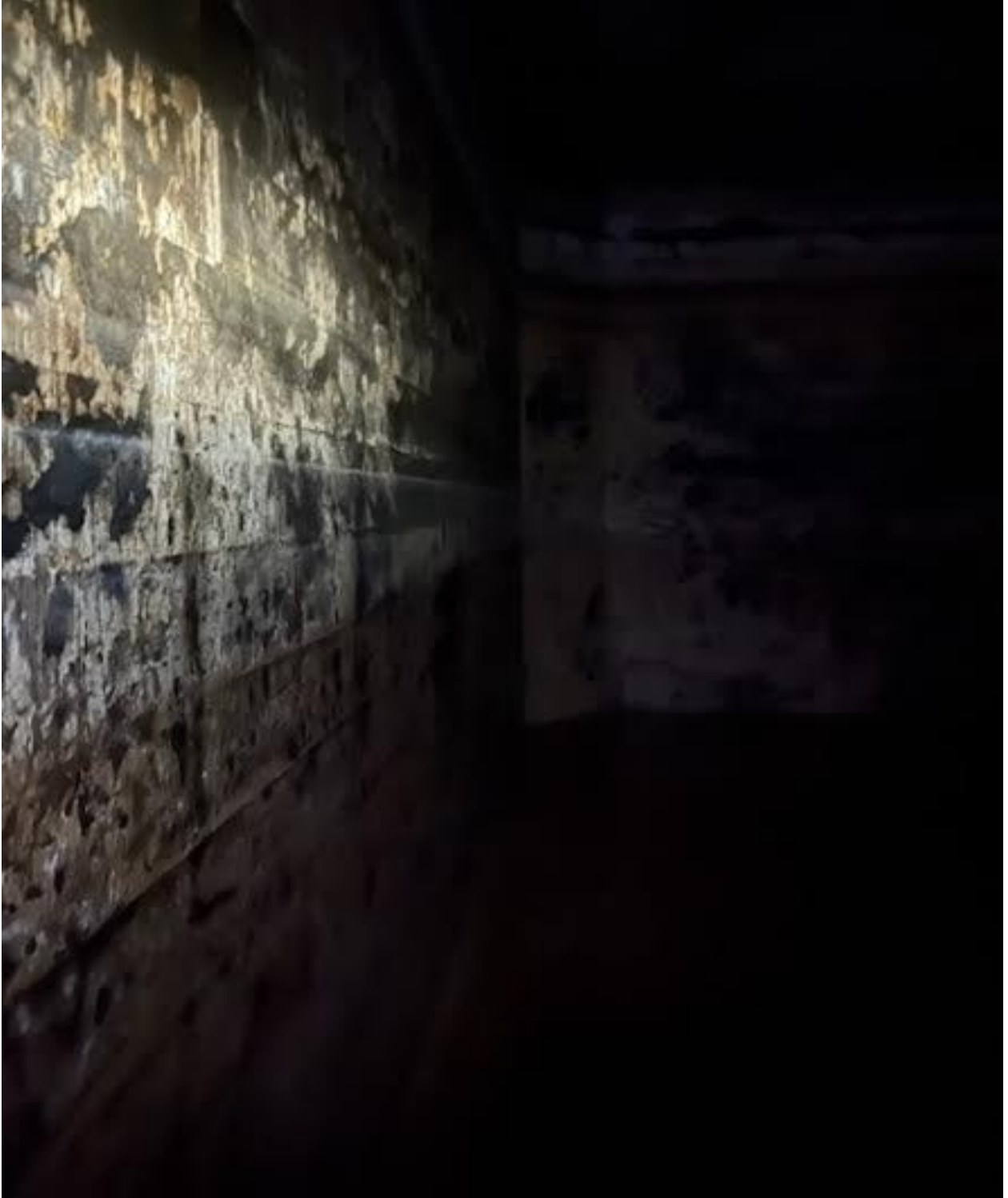
The Concrete Walls are in Good Condition
