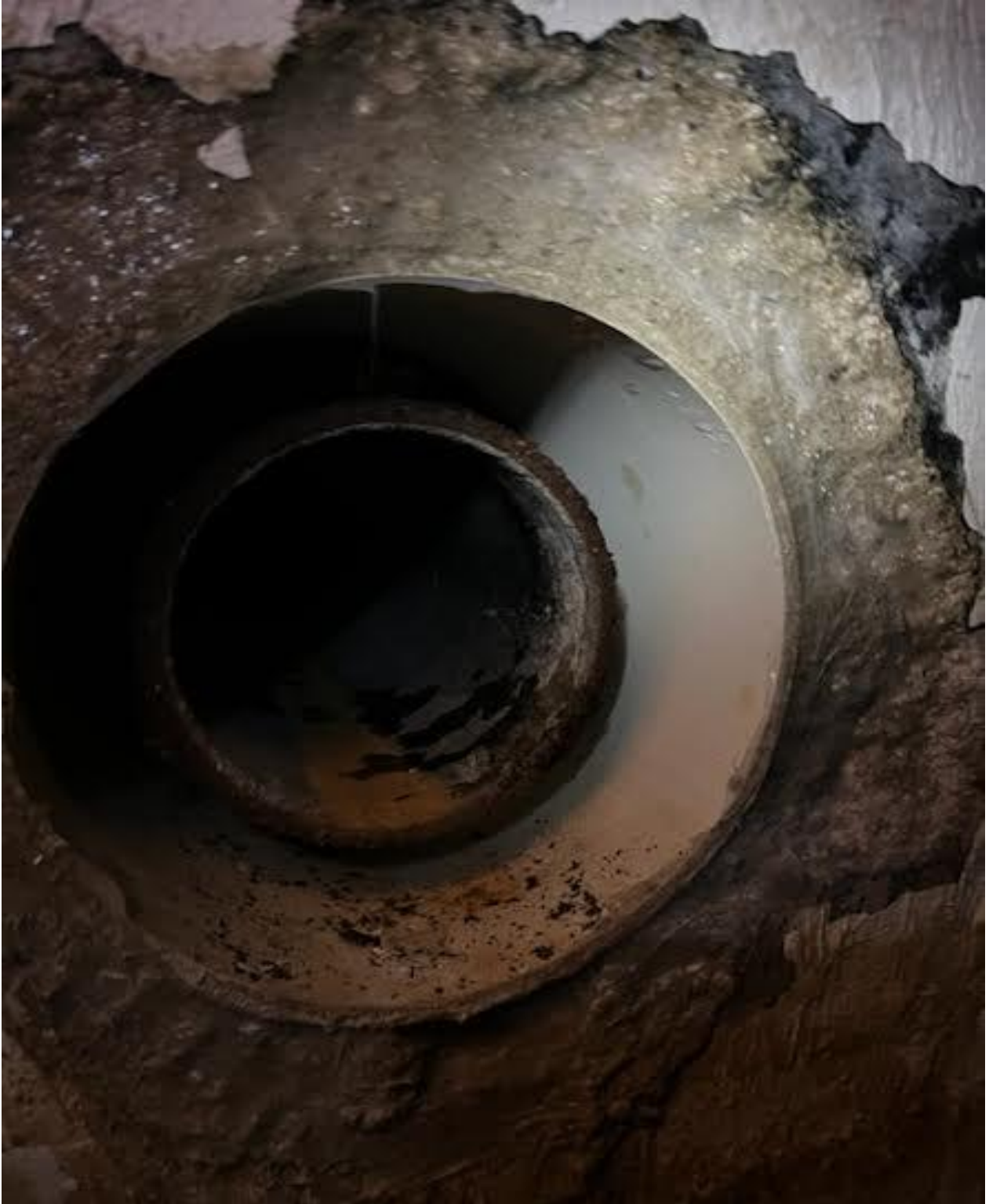
The Overflow Opening is in Good Condition
