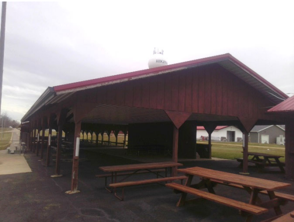
006005 - Picnic Shelter #3 (Exterior View)
