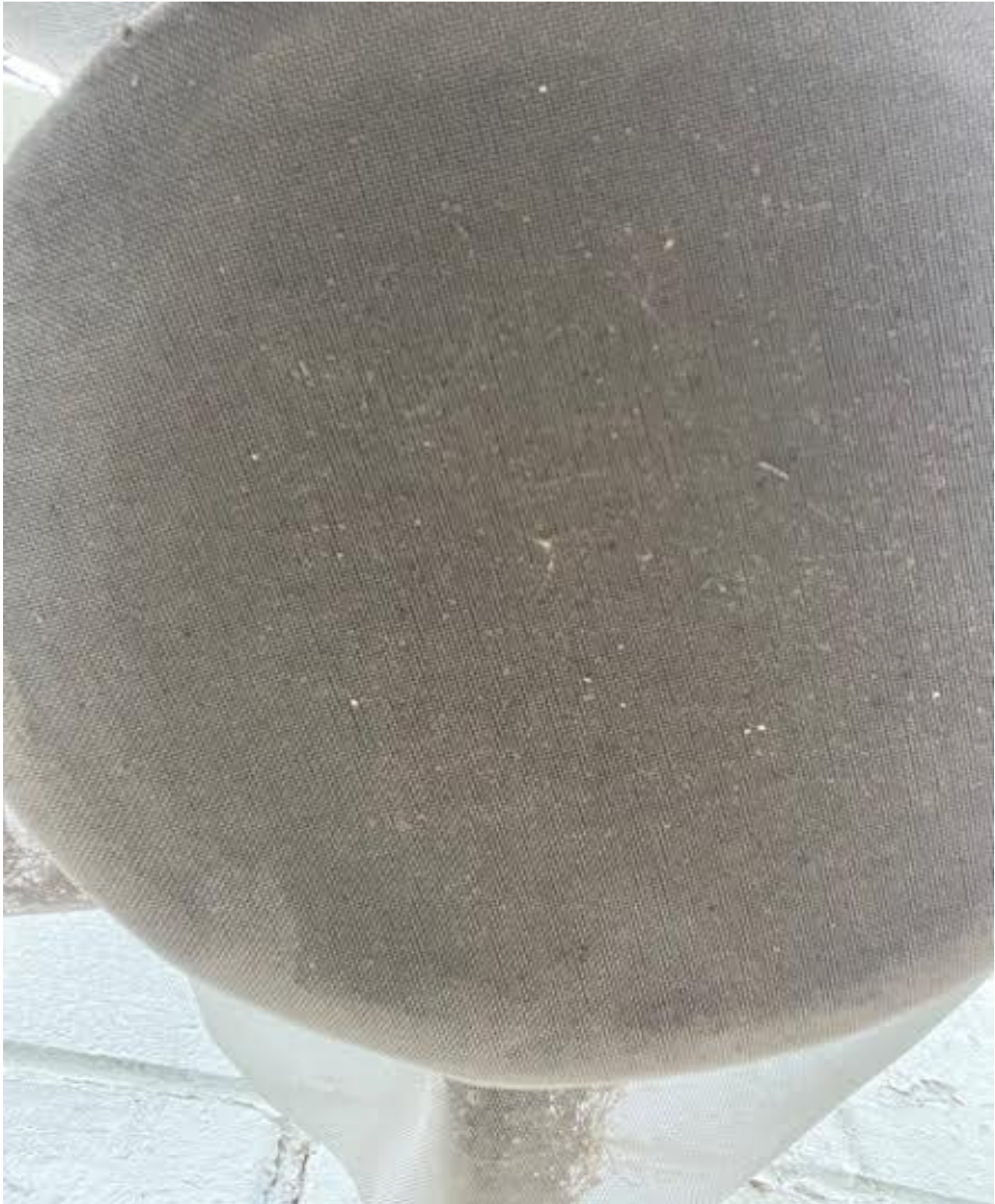
Overflow Screen is in Good Condition
