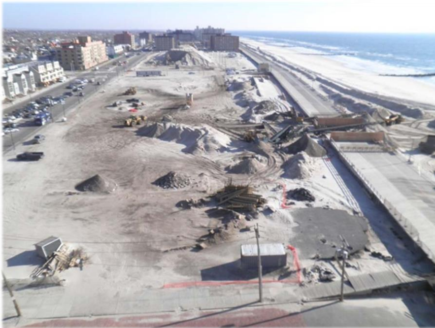
Sand Reclamation and Screening Site
