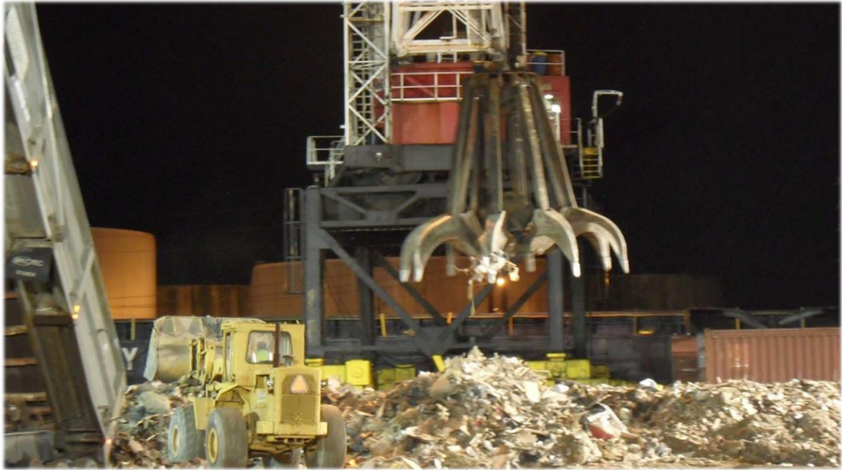
C&D Barging Site
