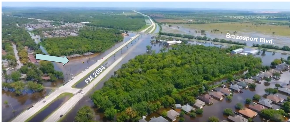
Hurricane Harvey drone flyover footage showing extensive flood damage.
