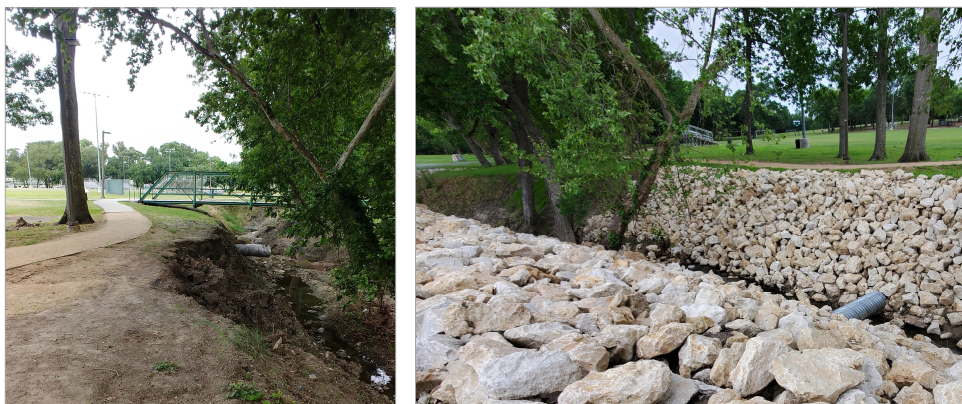
Hohlt Park before and after reconstruction of creek banks.
