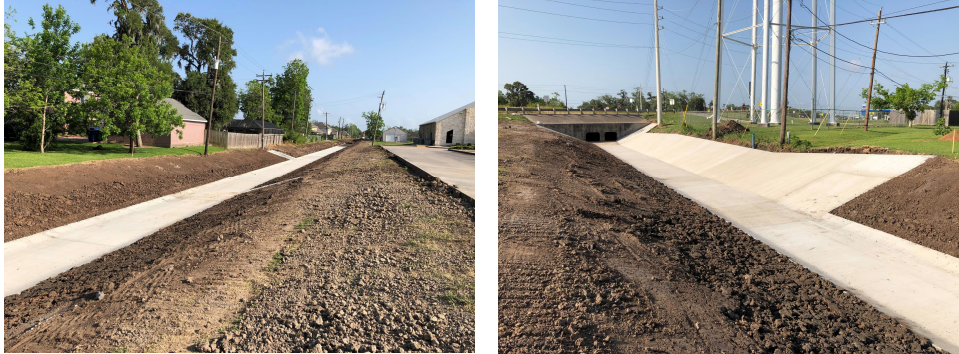
Construction of drainage improvements on the west side of the city.
