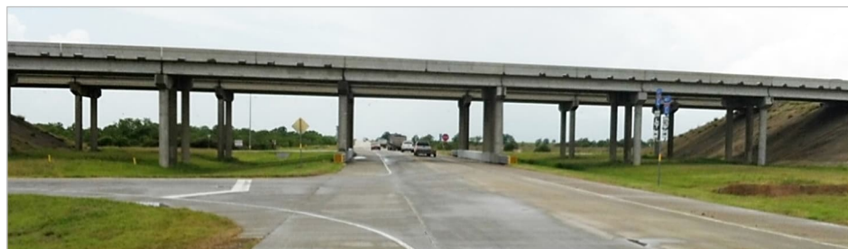
FM 3538 Roadway improvements to Walmart Distribution Center – Sealy, Texas.
