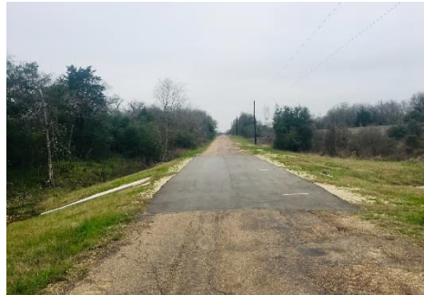
Completed concrete culvert and asphalt pavement repair.
