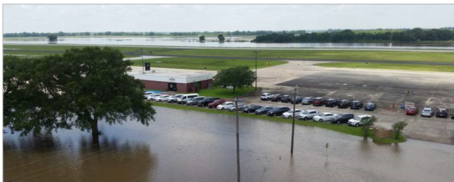
June 2016 flooding near the airport terminal building.
