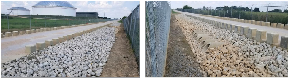
Reinforced roadway bed with multiple cross-drainage ports.
