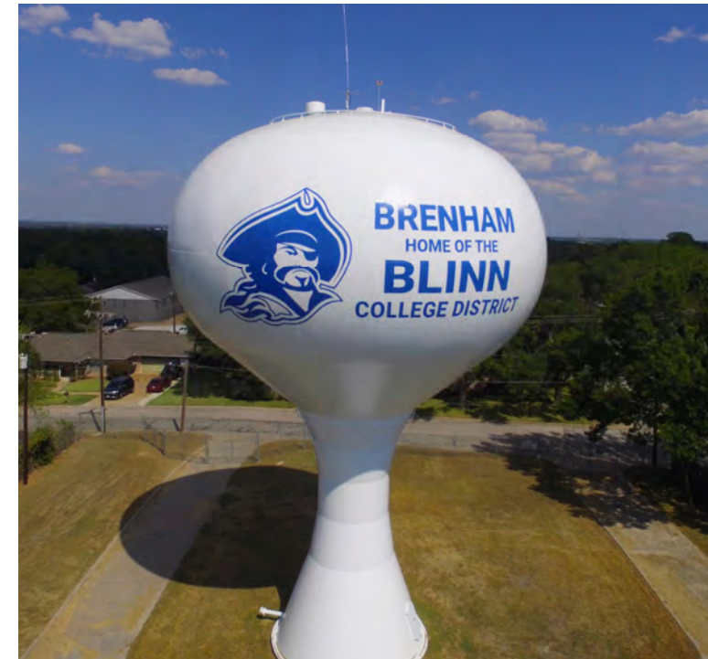
Atlow Elevated Storage Tank
