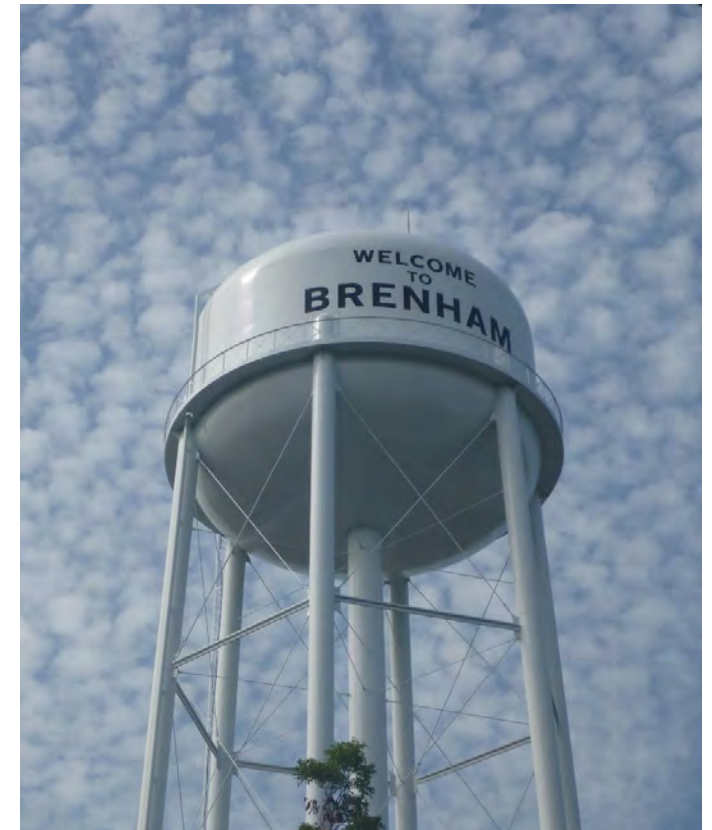
Church Street Elevated Storage Tank
