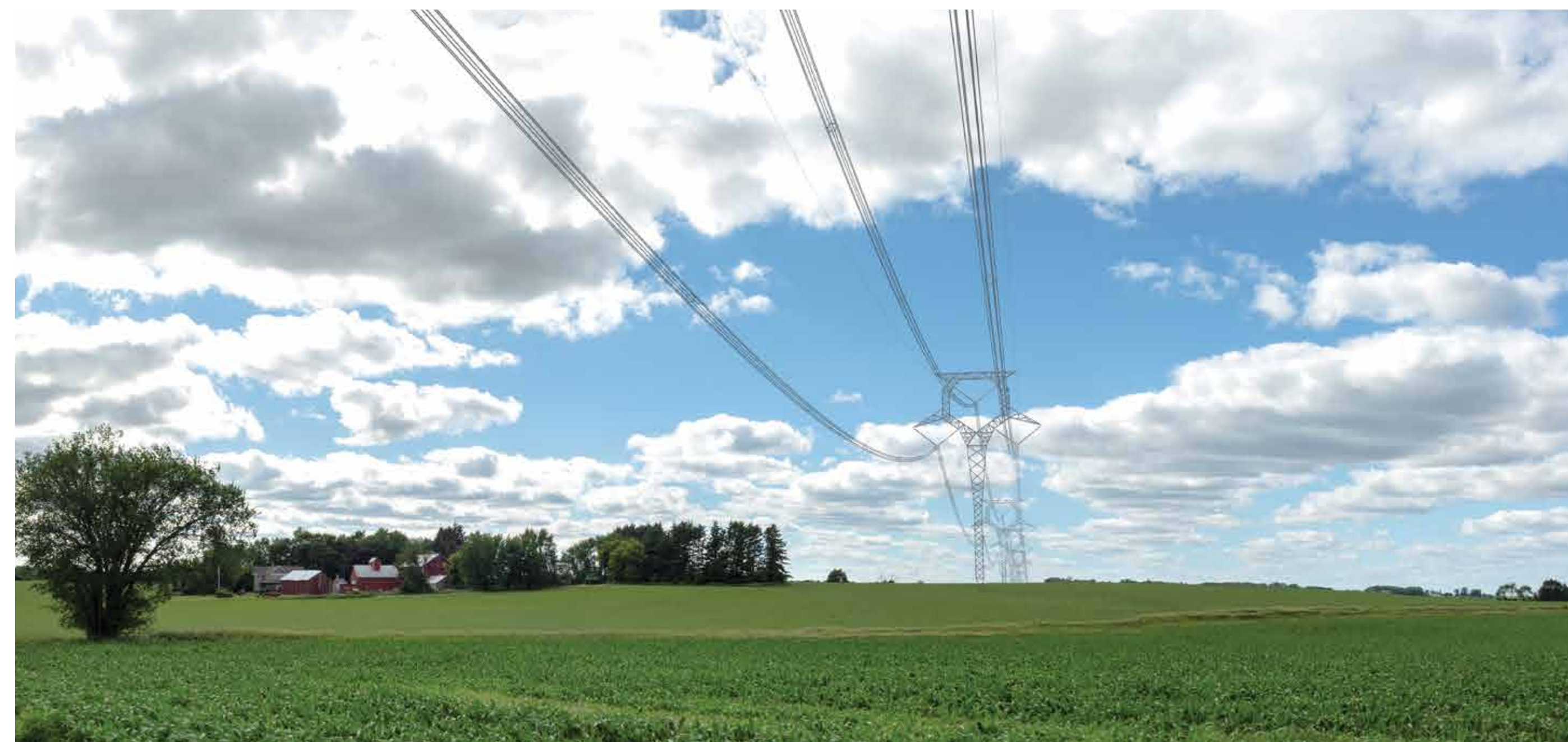
Structure heights are planned to support modern harvesting equipment.
