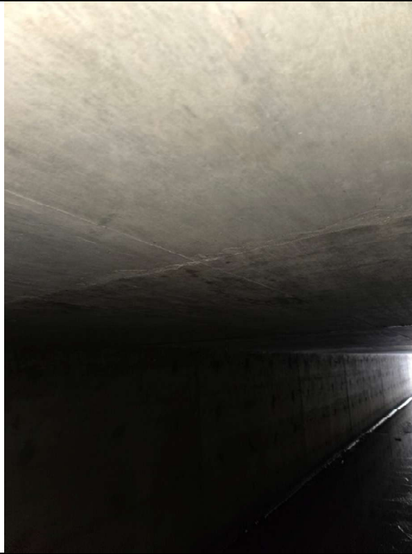
Photograph: 41 | Photo of concrete channel.
