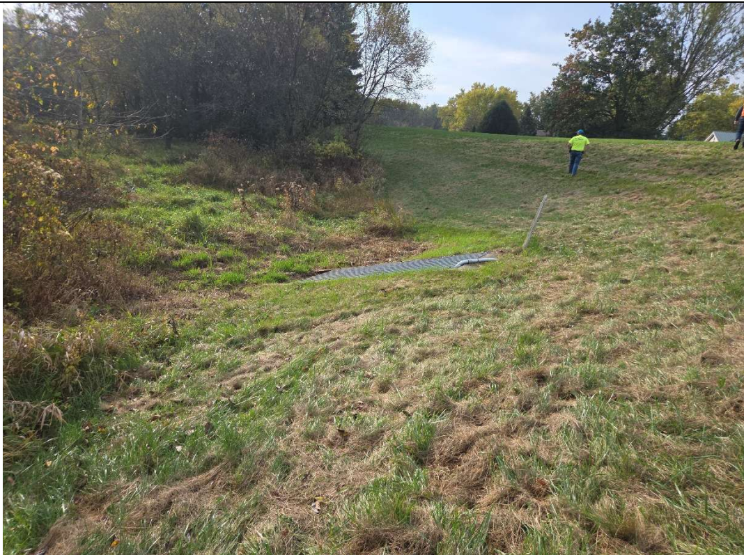
Photograph: 4 | Inlet and Valve at approximately Station 26+50.
