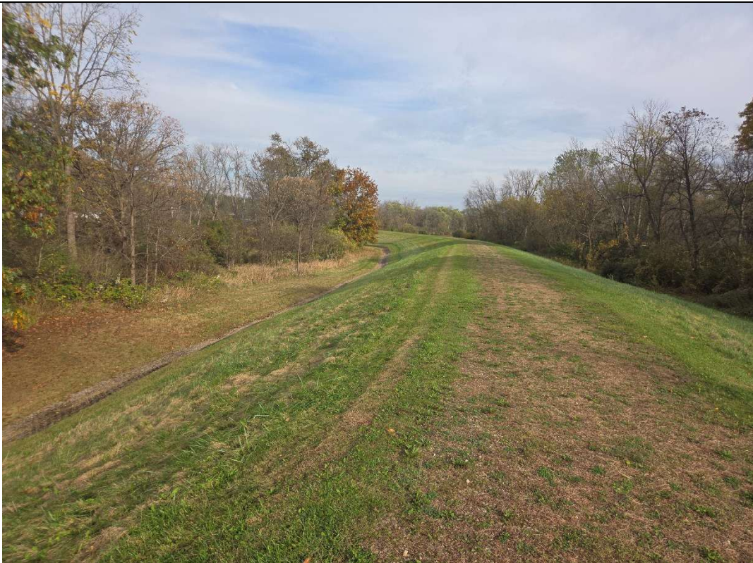
Photograph: 2 | Allison Park – general dike photo, viewing in Northerly direction.
