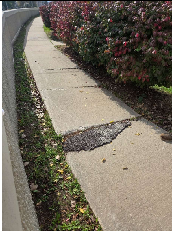
Photograph: 32 Photo taken of concrete dike viewing southerly to the west of N Congress Street.
