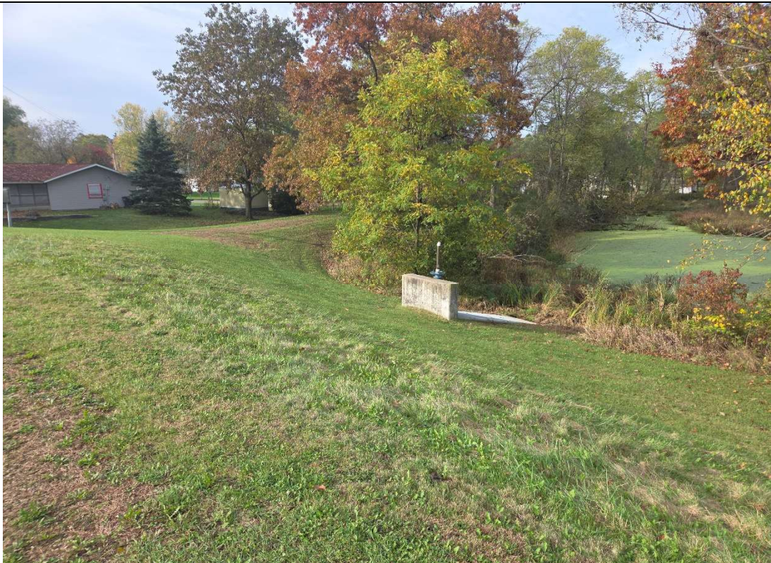
Photograph: 6 | Flood gate in good working condition.
