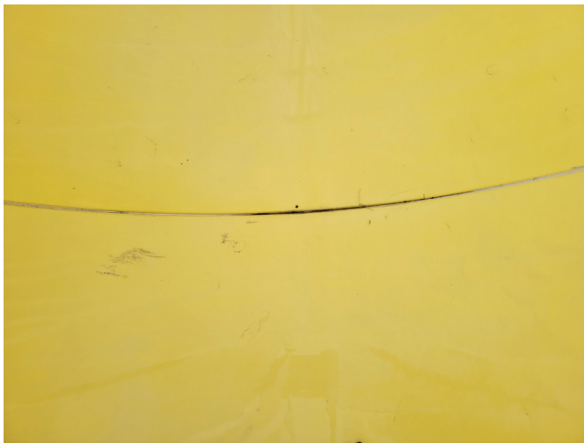
3. MISSING SEALANT
