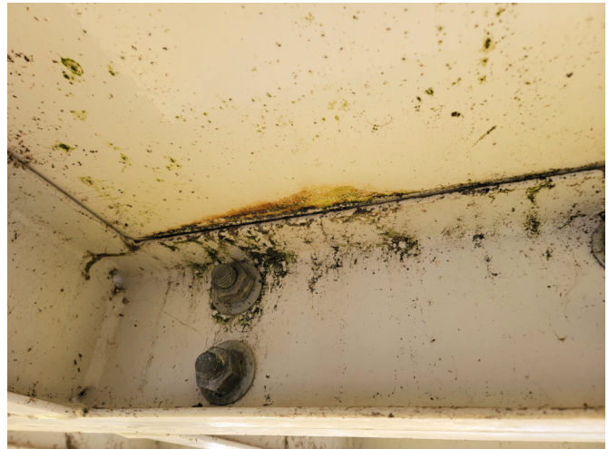
6. DIRT/ALGAE AND CORROSION UNDER PLATFORM
