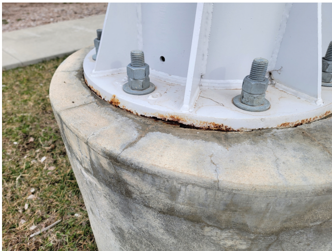
5. CORROSION ON BASE OF SLIDE SUPPORT
