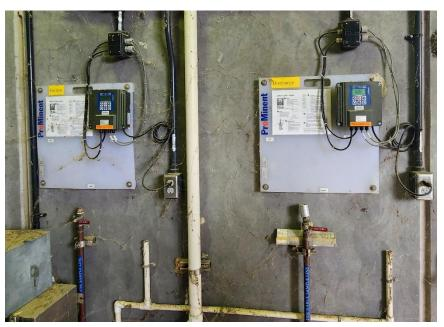
Figure 2-5: Chlorine Analyzer Controllers
