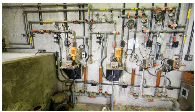
Figure 2-4: Sodium Hypochlorite and LAS Metering Pumps
