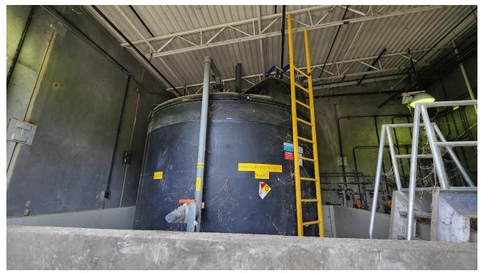
Figure 2-1: Bulk Sodium Hypochlorite Tank
