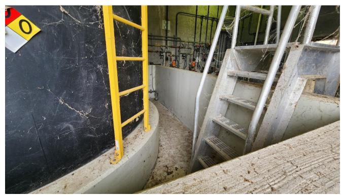
Figure 2-2: Bulk Sodium Hypochlorite Containment Area
