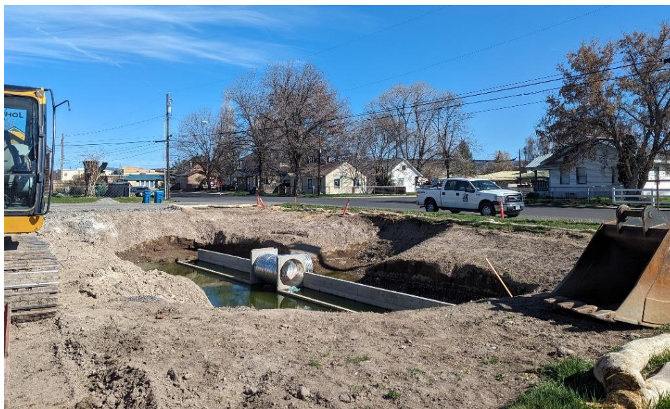
Stormwater improvements continued during the fourth quarter.
