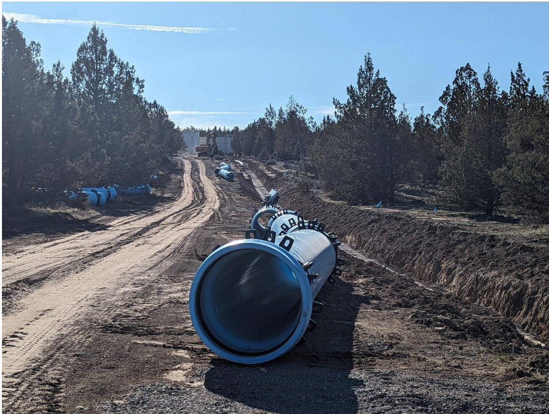
Pipe ready to be installed for the waterline extension project in the fourth quarter.
