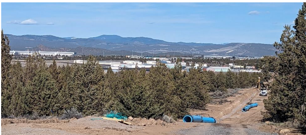
Waterline extension project work during the fourth quarter.
