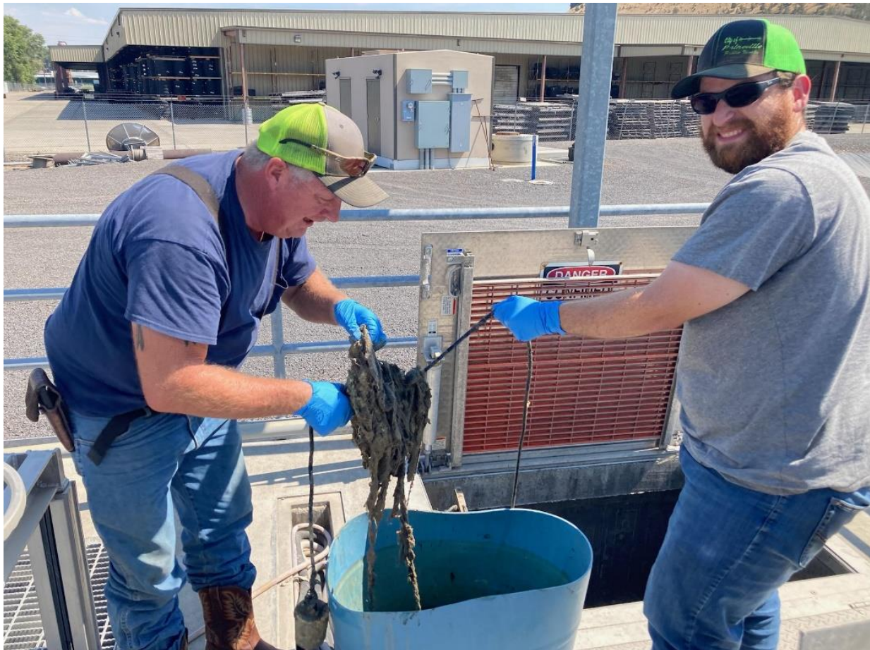
Wastewater Treatment Plant Screens being cleaned by staff in July 2022
