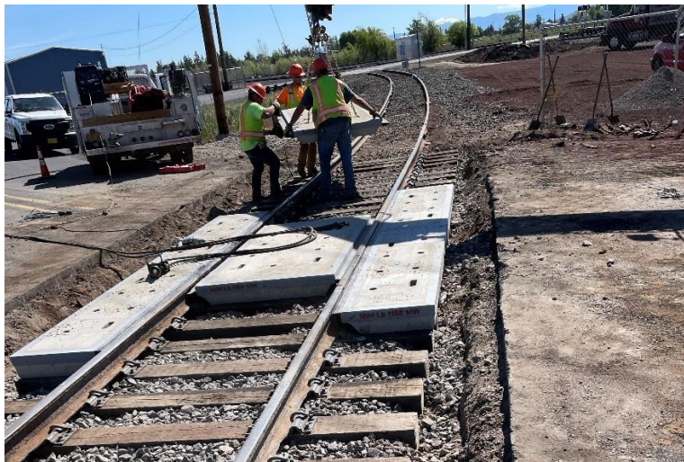
Public Works helped the railroad with crossing work completed in the first quarter.
