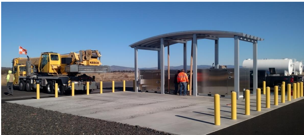
New fuel system, which is partially funded through a Connect Oregon grant, being installed at the airport during the first quarter.
