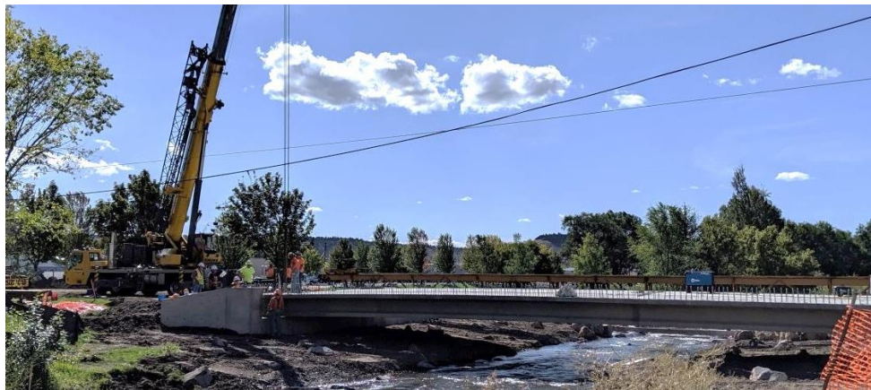
Construction of the Elm Street Bridge during the first quarter.
