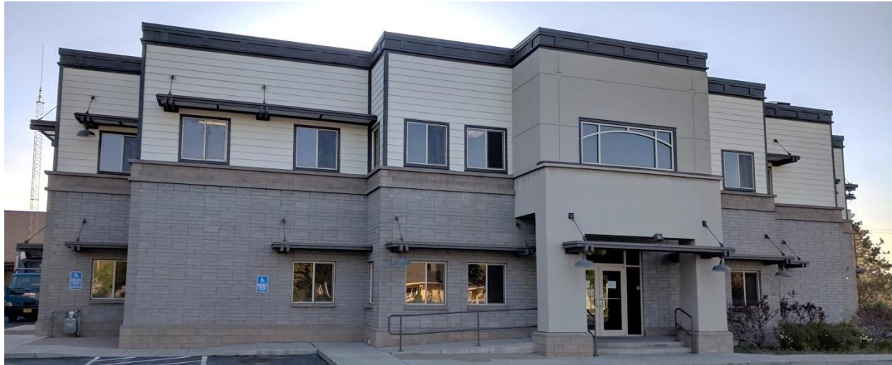
The new Police Facility building (pictured above) that was purchased during the fourth quarter.
