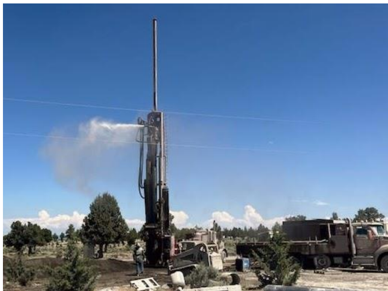
Well work being done in July 2025.
