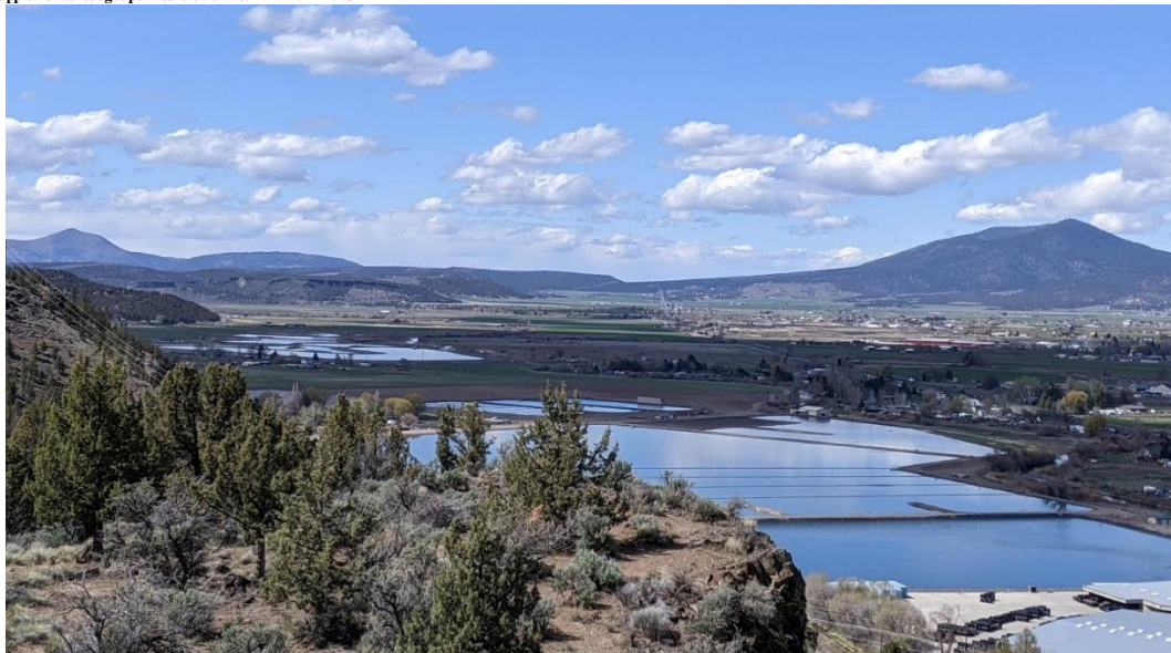
Wastewater treatment facility in April of 2022.
