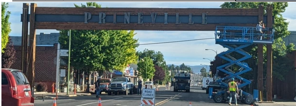
New downtown arch being installed on 6/30/22.
