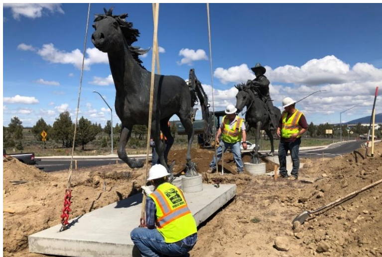
Public Works installing the artwork for the roundabout in June of 2022.
