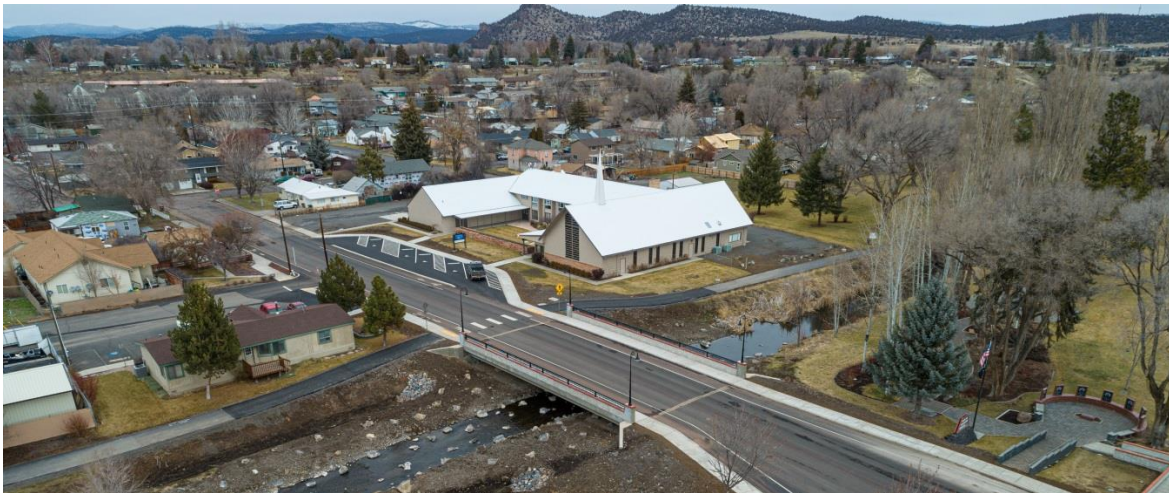
Drone photos taken of the new Elm Street Bridge in January 2020.
