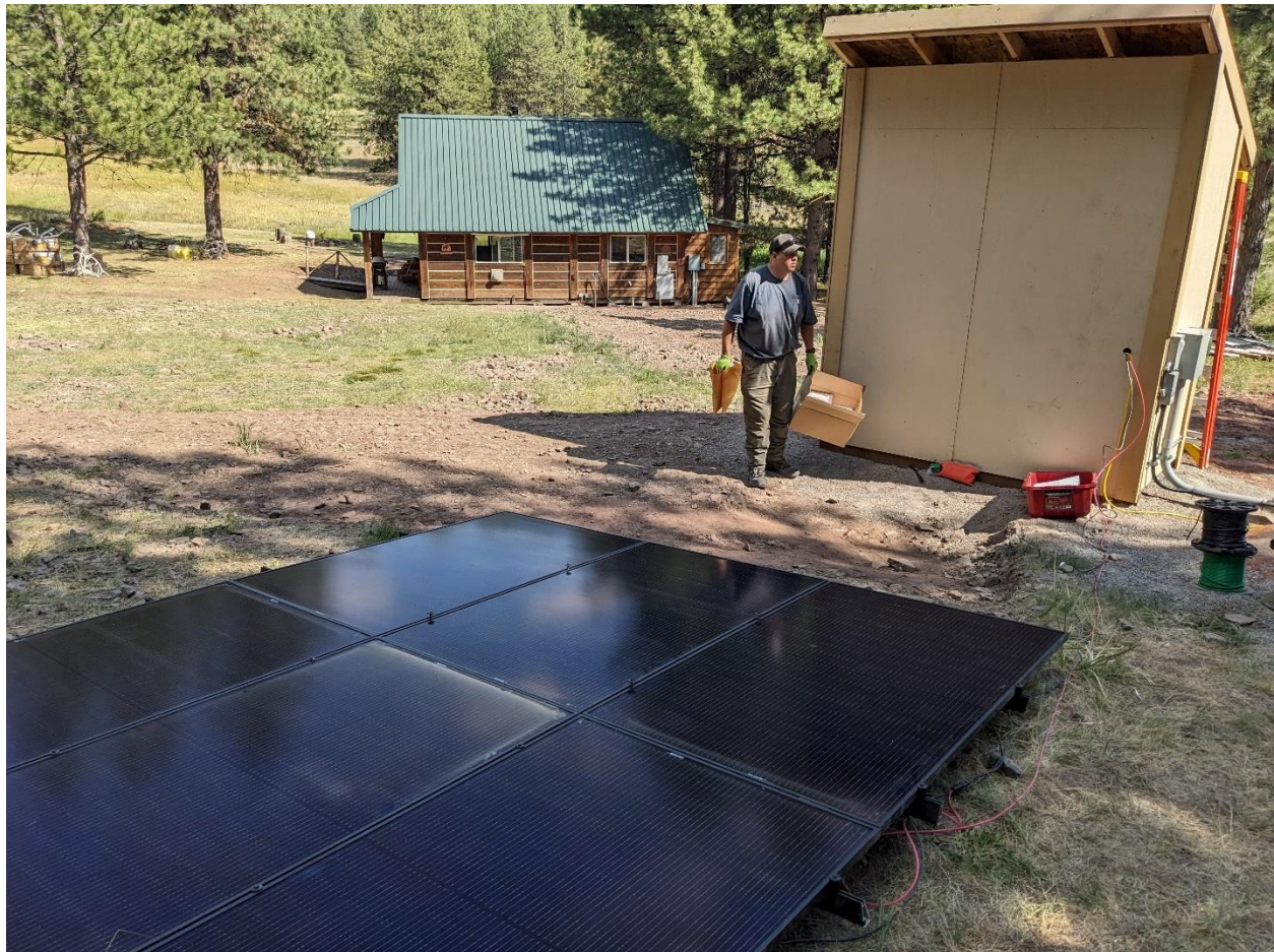
IT work being done during July of 2023
