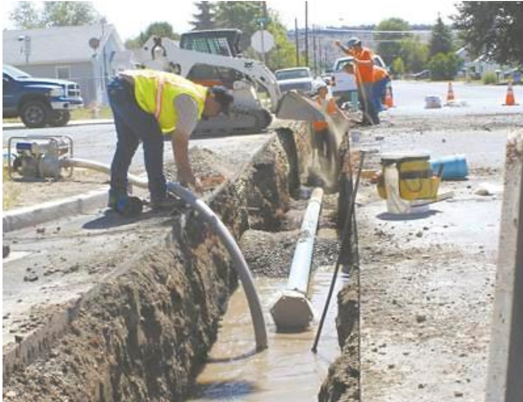
Photo taken by Jason Chaney of the Central Oregonian as the last wooden water line was removed during the first quarter.
