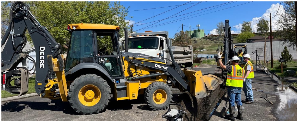
The Dunham waterline project in August 2023
