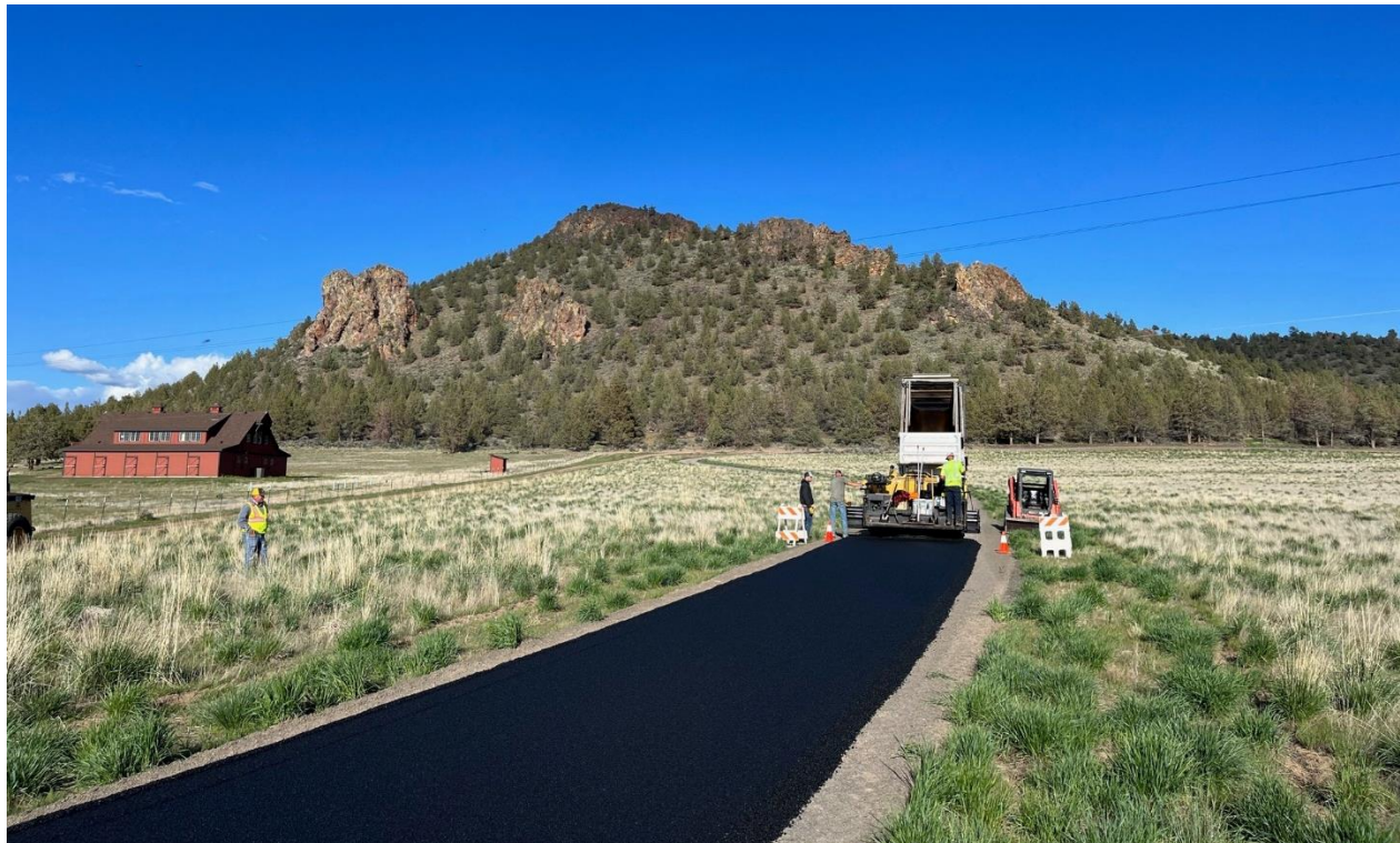
Trail paving work continued through the third quarter at Barnes Butte
