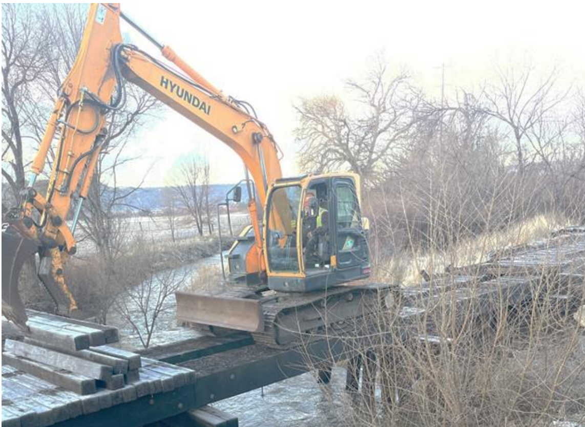
Bridge work being done during the third quarter.
