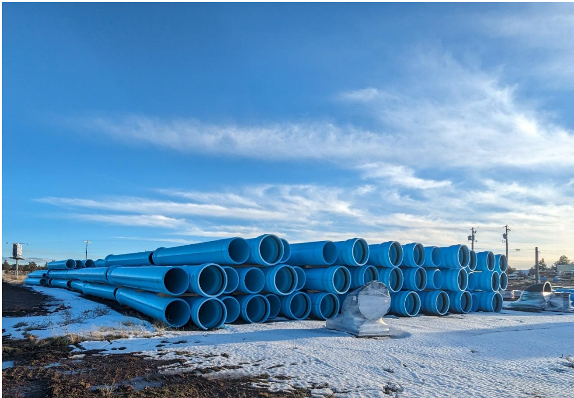
Pipe ready to be installed for the waterline extension project in the third quarter.
