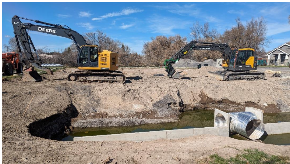
Stormwater improvements being made in March 2024.
