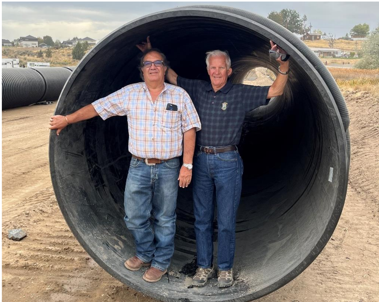
Steve Forrester (City Manager) and Steve Uffelman (City Councilor) inspecting the pipe being used for the canal in the Combs Flat project.
