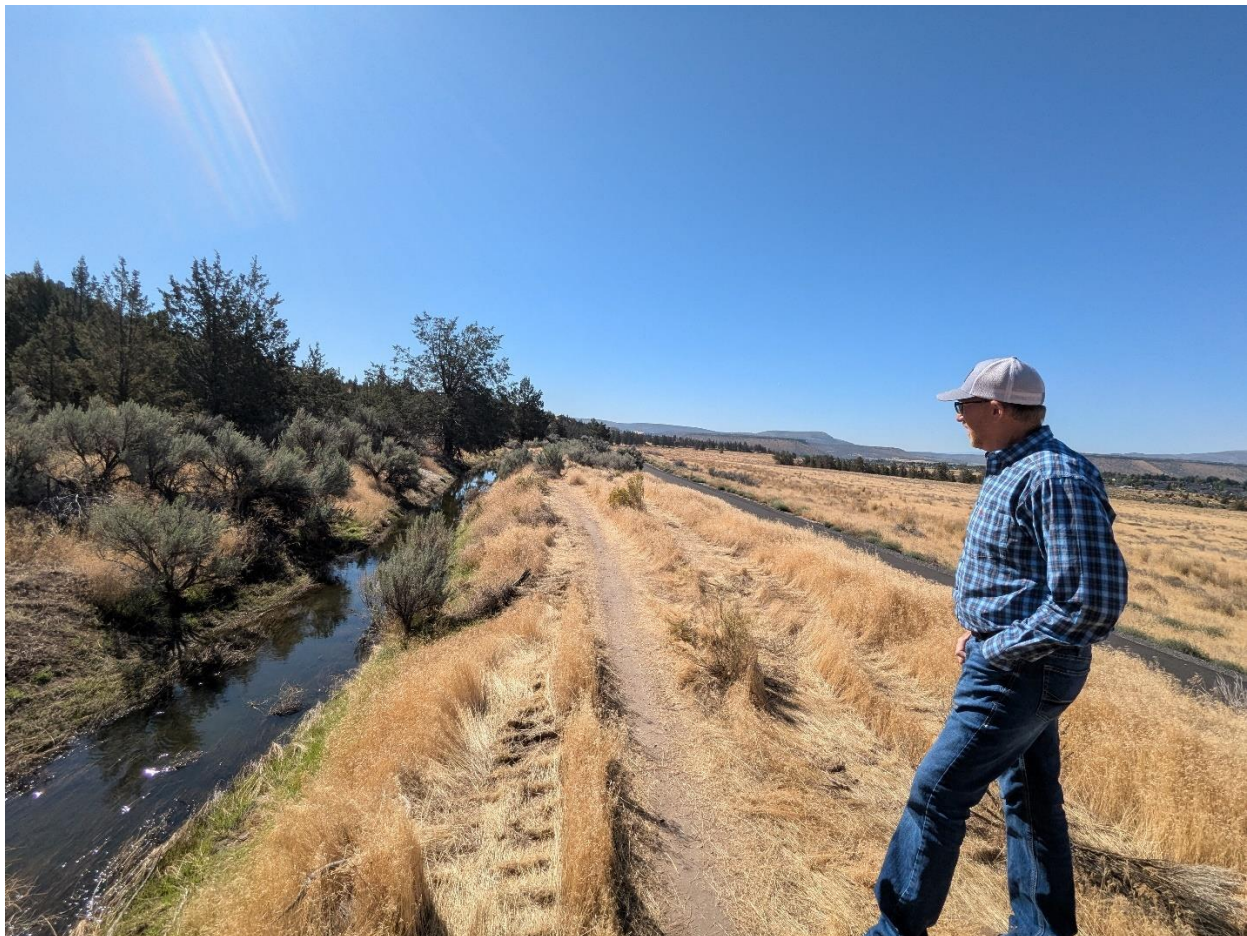
PW Director / Assistant City Manager, Casey Kaiser, inspecting the renewed canal at BBRA during the first quarter.
