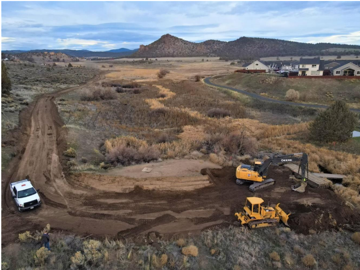
Pedestrian bridge being installed for additional access to Barnes Butte.
