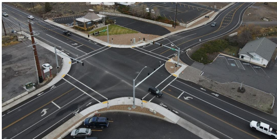
Completed 10 th and Main realignment – pic taken in November 2021
