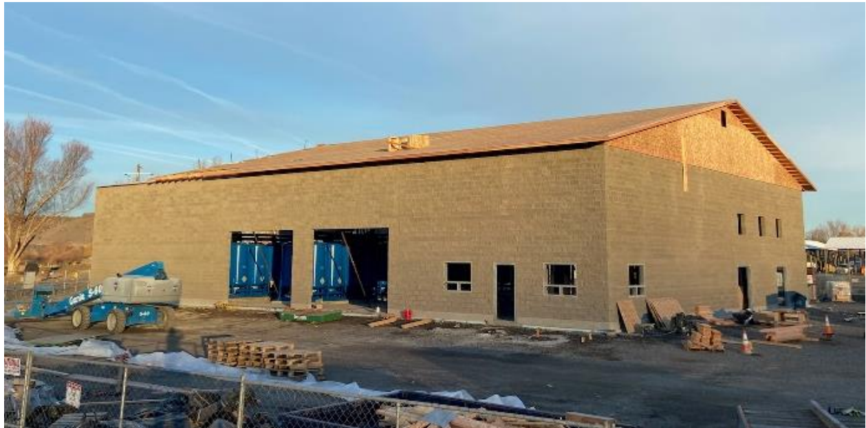
Second quarter progress of the ASR building.
