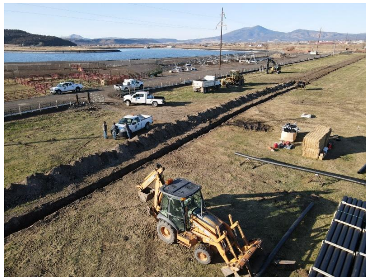
Irrigation upgrades being done at the WWTP during the second quarter.
