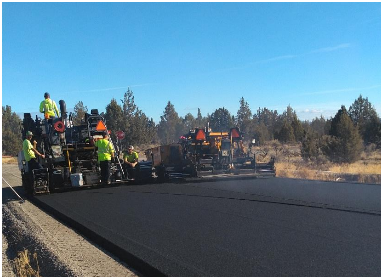
Helibase paving at the airport that took place during the second quarter.
