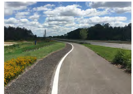
A dual surface trail could provide opportunity for a variety of user types. Bexley, OH
