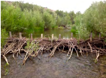
In Oregon's Bridge Creek Watershed, researchers built a number of beaver dam analogs to encourage increased beaver activity and restore river habitat. Credit, Utah State University
