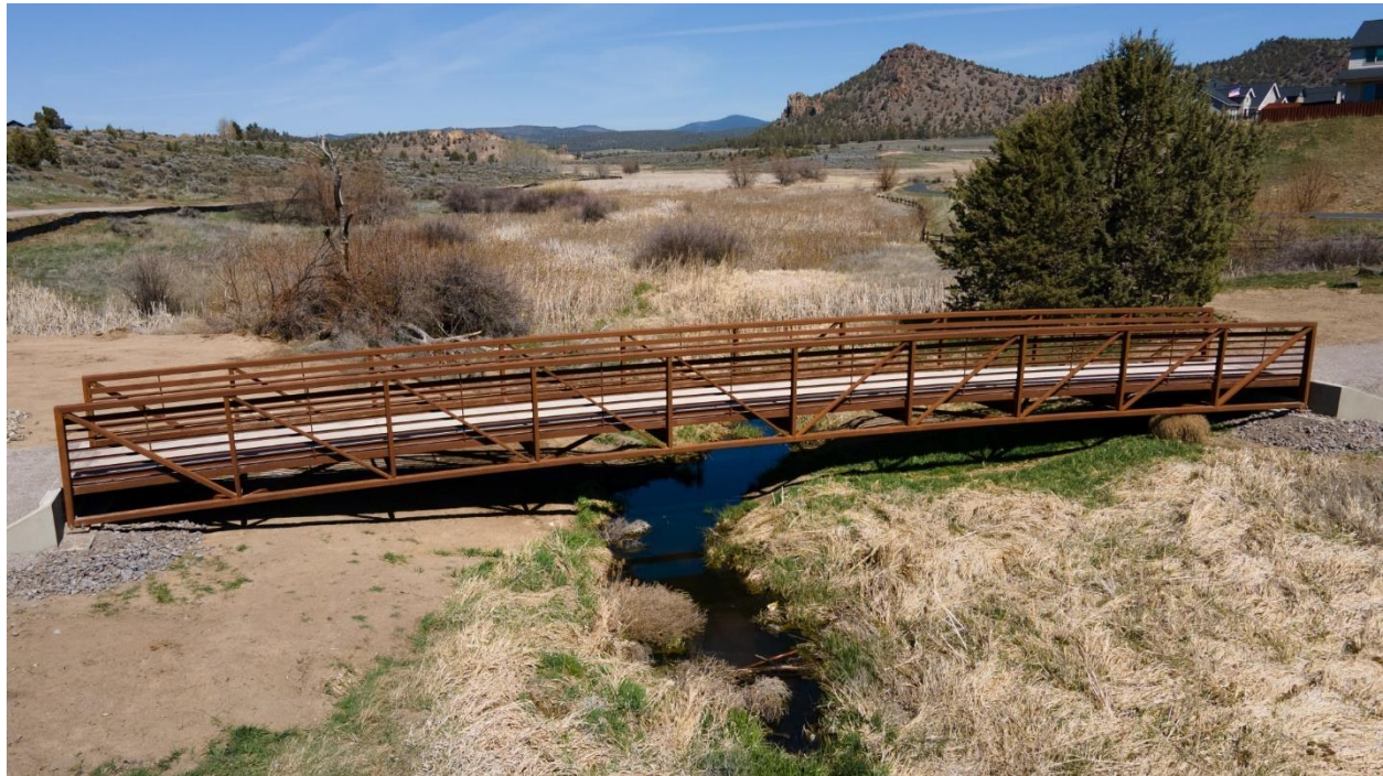
Pedestrian bridge completed during the third quarter for additional access to Barnes Butte.
