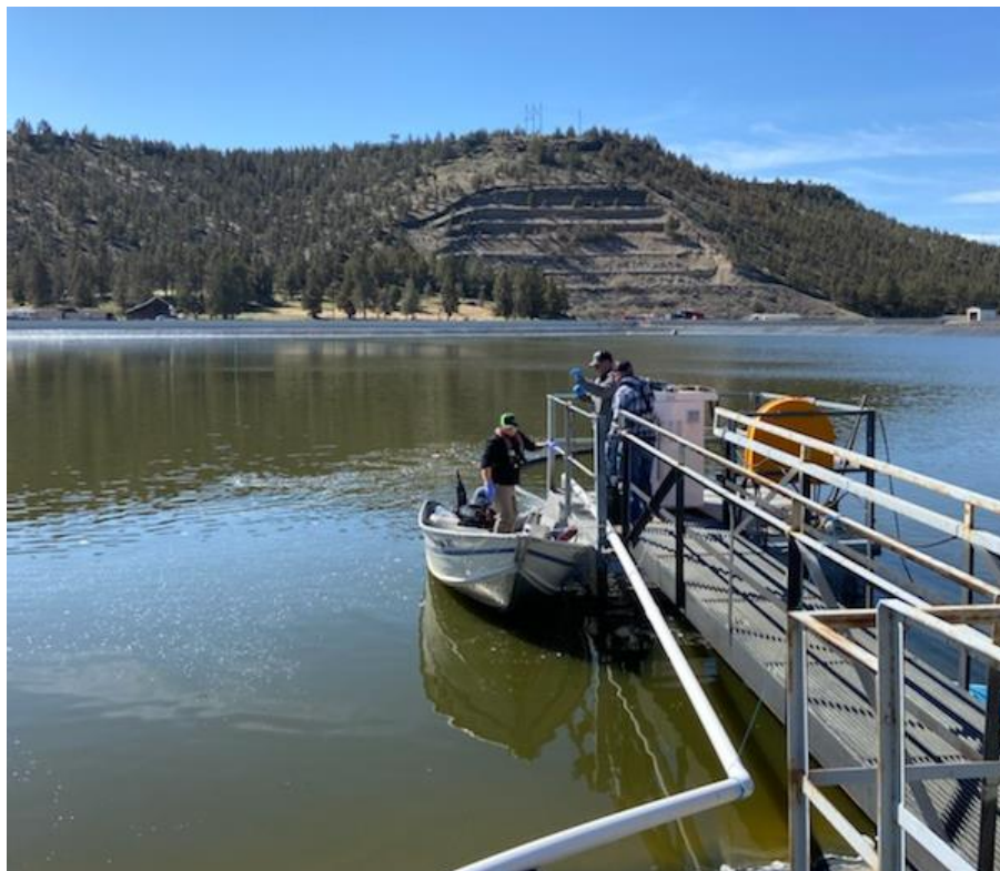
Wastewater crew getting ready to do some pump repairs in March 2022.
