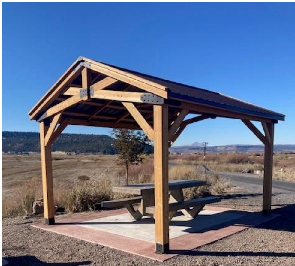
New Gazebo built at the wetlands during the second quarter.
