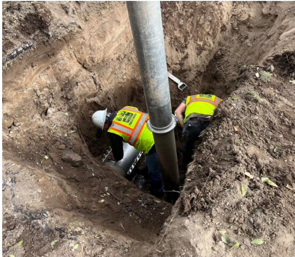
Utility line work being done during the second quarter.
