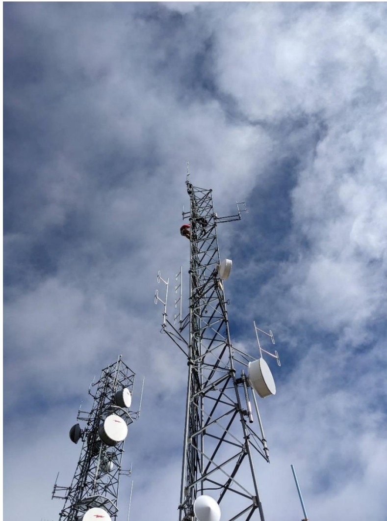
Tower work being done by IT during October of 2023
