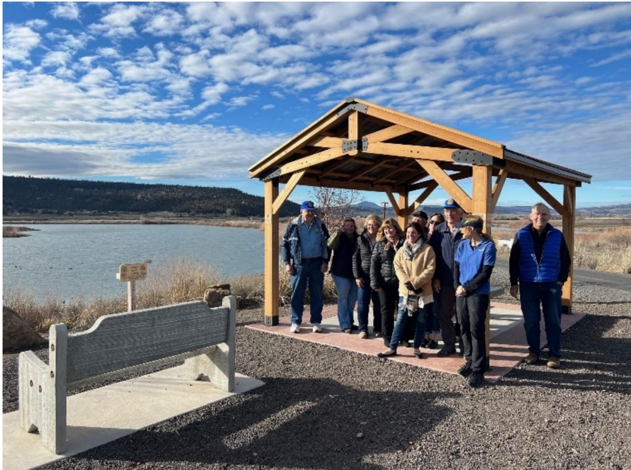
New Gazebo built by PW at the wetlands during the second quarter.
