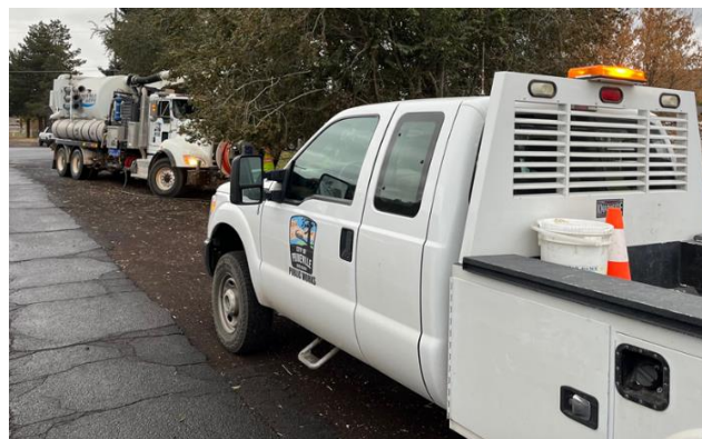
Utility work being completed during the second quarter.
