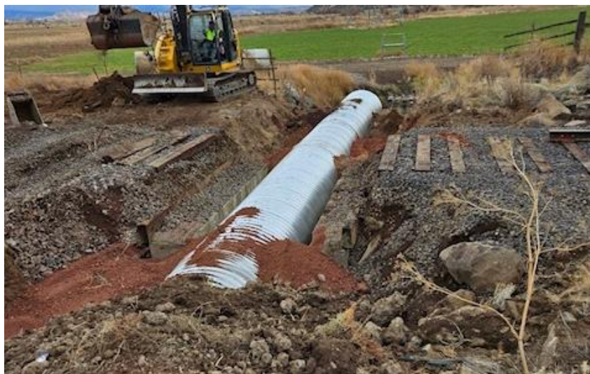
Lytle Creek bridge was removed and the creek was piped in November 2024.
