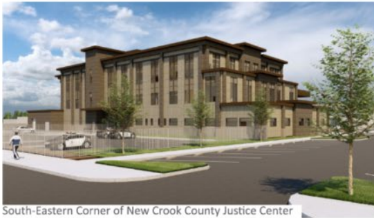
South-Eastern Corner of New Crook County Justice Center
