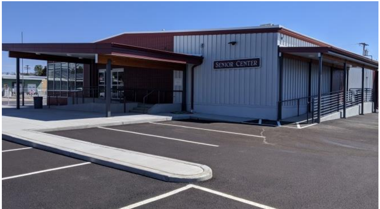
The Sr. Center project near completion during the first quarter.
